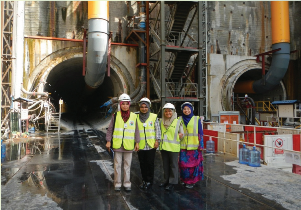
Gambar3(b): Pembinaan Mass Rapid Transit Tunnel
