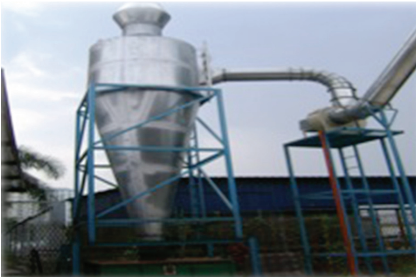
Alat kawalan pencemaran udara cyclone dust collector
