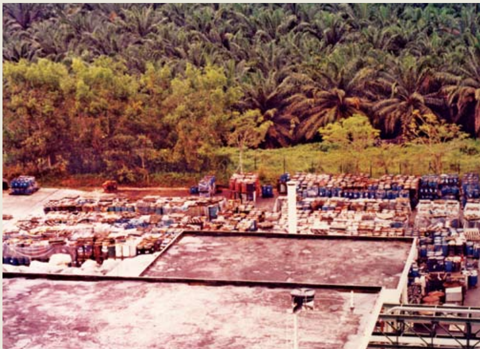
Aerial view of storage facility at the Integrated Toxic and Hazardous Wastes Facility
