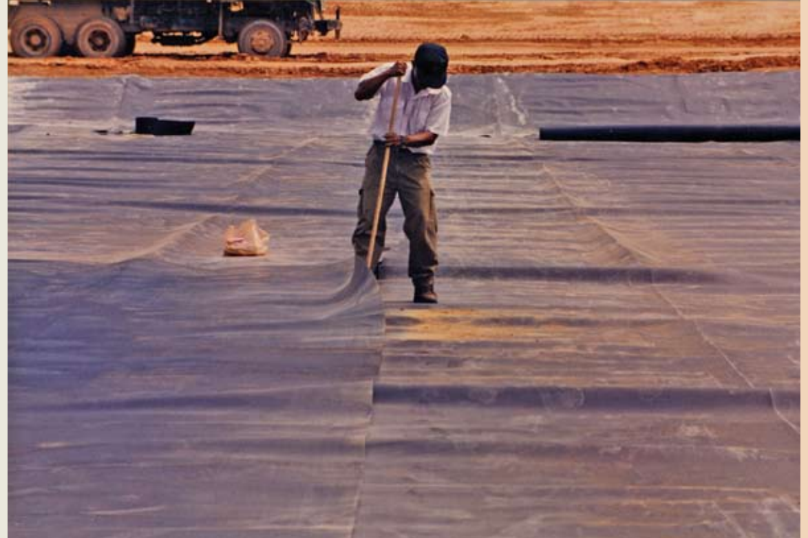
Installation of liners at a secured landfill
