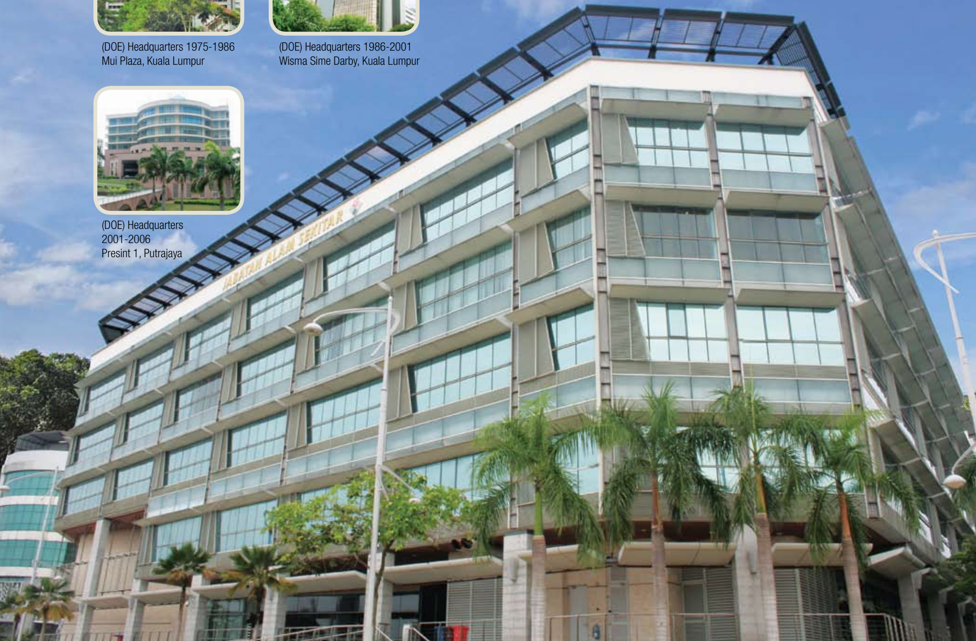
Department of the Environment (DOE) Headquarters in Presint 4 Putrajaya, 2010
