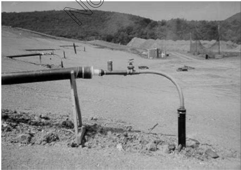
Figure A.5. Horizontal LFG extraction well
