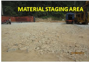
Gravelling BMPs of rutted access road
