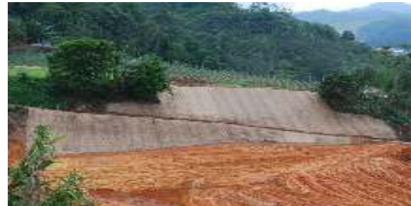
Slope Formation Stabilization Mat: 16.4.2009
