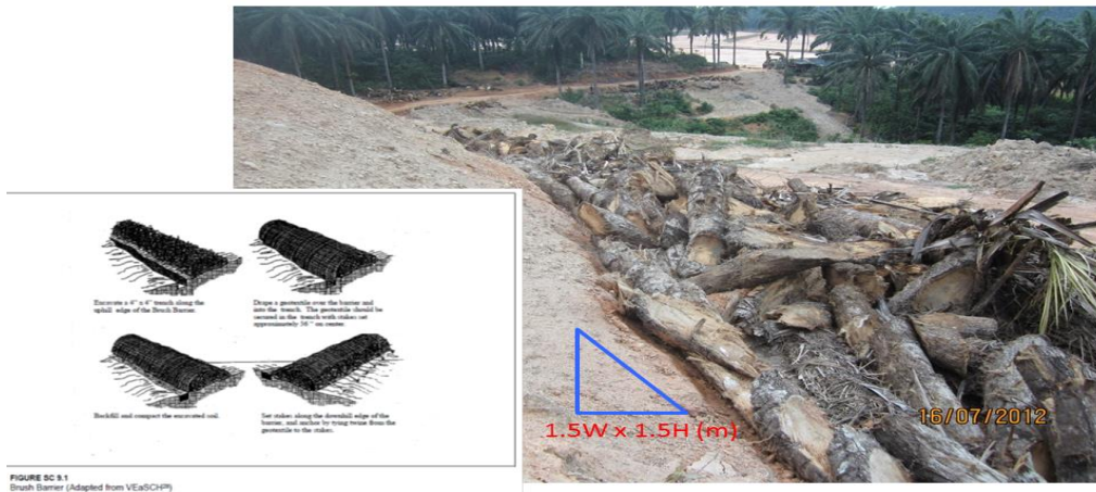
FIGURE DC 8.1 Brush Barrier (Adapted from VEA/SCHP)
