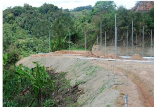
PLOT 6: SLOPE STABILIZATION 30.4.2009
