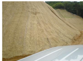
PLOT 11 SLOPE STABILIZATION:26.5.2009
