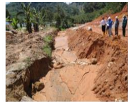
SILTED CHECK DAM (DRY)
