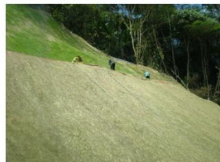
PLOT 11 SLOPE STABILIZATION: 1.6.2009
