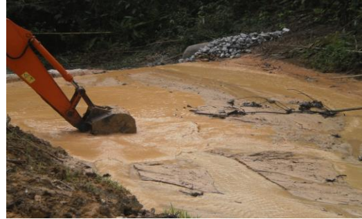
iv. Maintenance in progress
