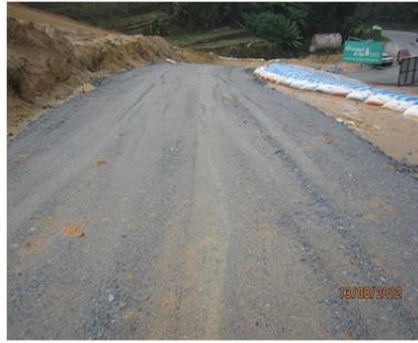
Gravelling BMPs of rutted access road
