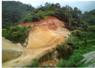
PLOT 11 SLOPE STABILIZATION: 11.5.2009
