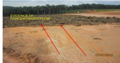
Potential to wash away due to less coverage
