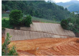
Slope Formation Stabilization Mat: 16.4.2009
