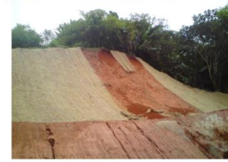
PLOT 11 SLOPE STABILIZATION: 14.5.2009
