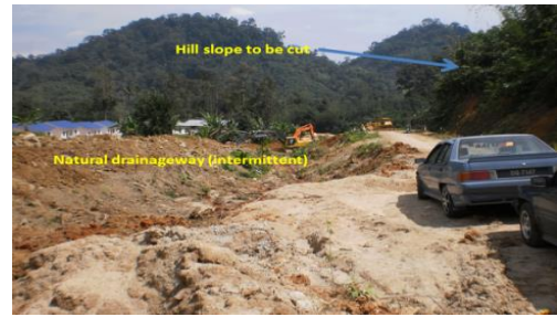
Establish road ditch / channel for runoff conveyances
