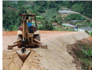
PLOT 6: PERIMETER EARTH (should construct before installations of blanket) DRAIN 14.4.2009
