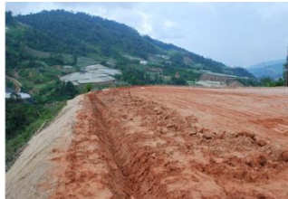
PLOT 6: PERIMETER EARTH DRAIN 16.4.2009
