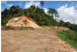
PLOT 8 SLOPE STABILIZATION: 29.4.2009
