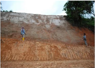
Slope Formation Hydroseeding: 15.4.2009
