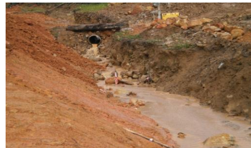
Install Check Dam
