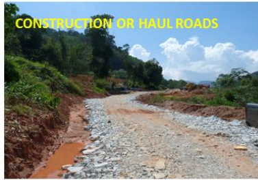
Gravelling BMPs of rutted access road
