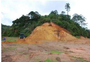
PLOT 8 SLOPE STABILIZATION: 2.5.2009
