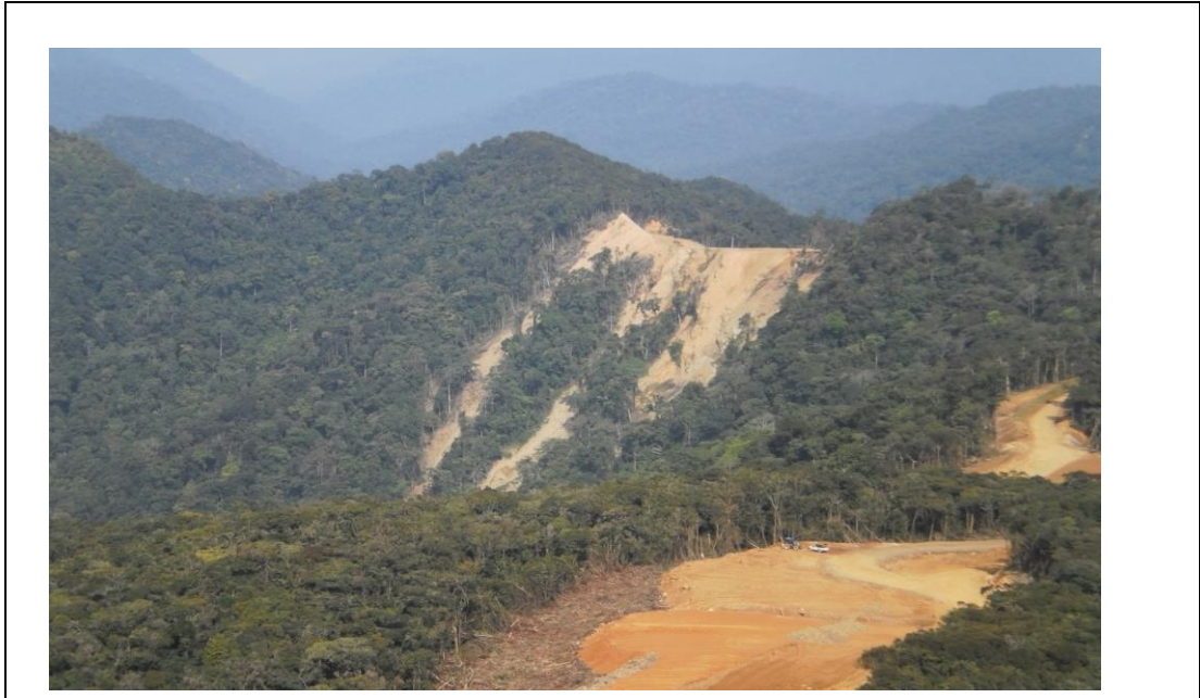
Figure 4.9: Erosion and Landslides Resulted from Lack of Activities Phasing
