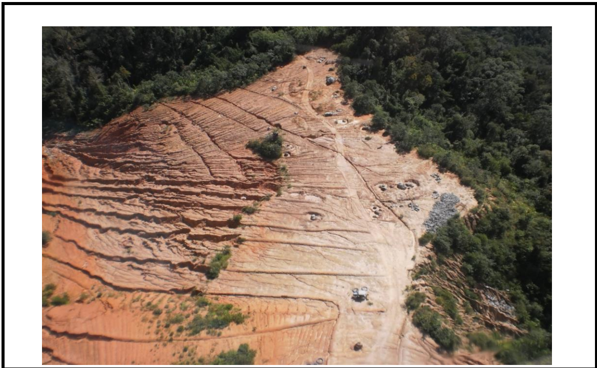
Figure 4.4: Vast Land Clearing with Lack of Phasing Planning
