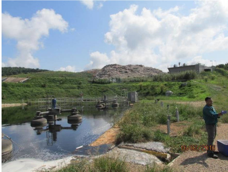
LOJI RAWATAN LEACHATE, TAPAK PELUPUSAN SAMPAH LADANG CEP RENGAM
