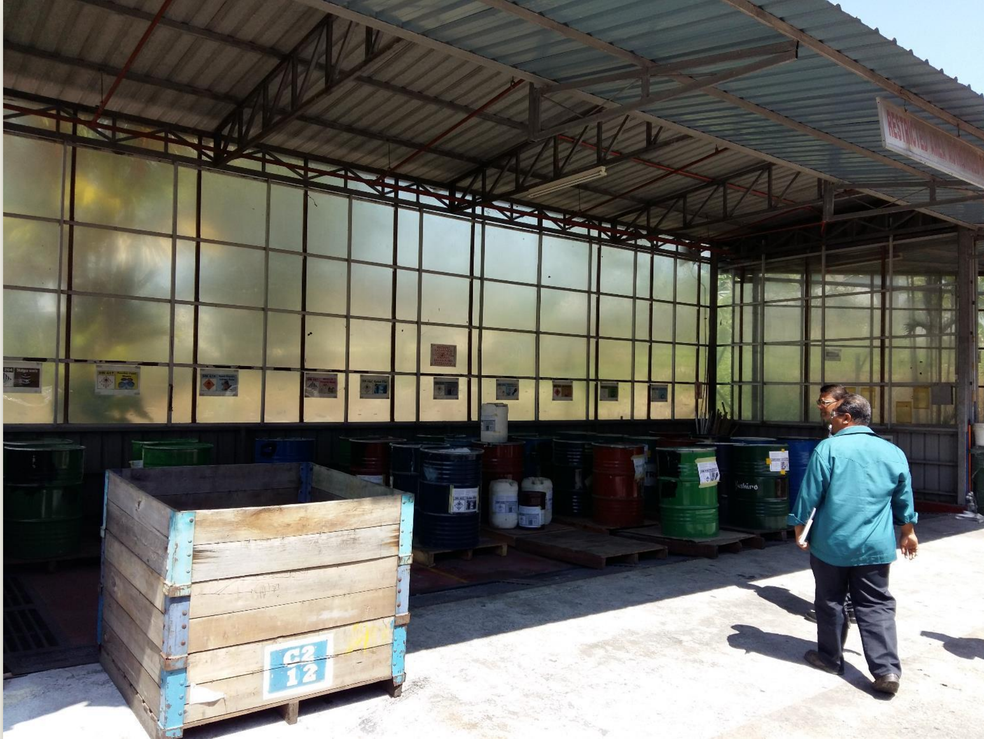
The scheduled waste storage at EMERSON.
