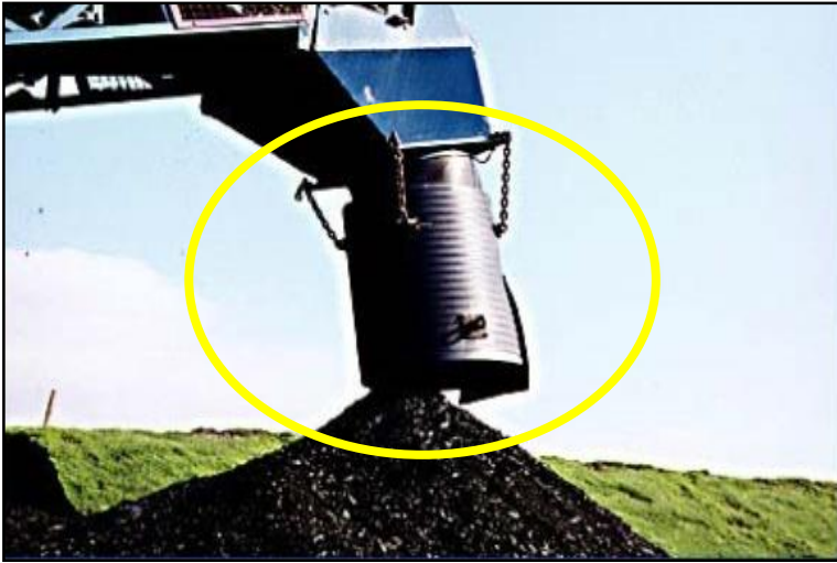
Sleeve on end of conveyer to reduce apparent drop height
