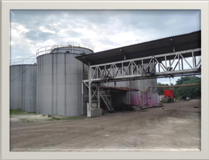
CPO STORAGE TANK
