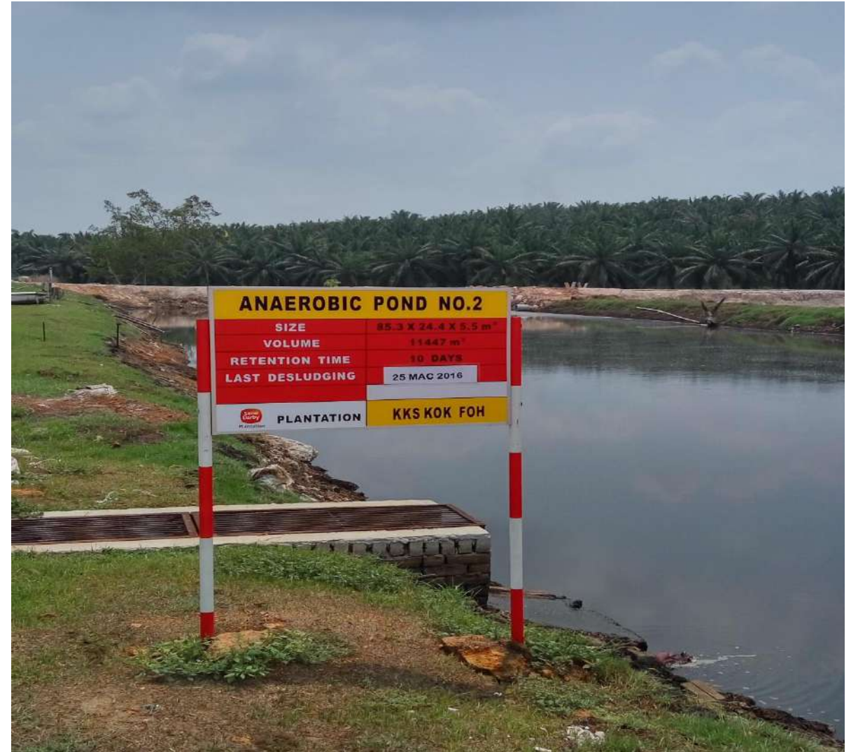
ANAEROBIC POND NO.2
