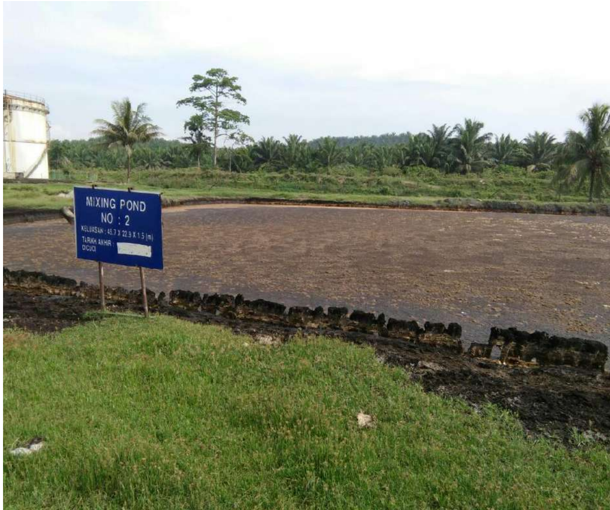
MIXING POND NO. 2
