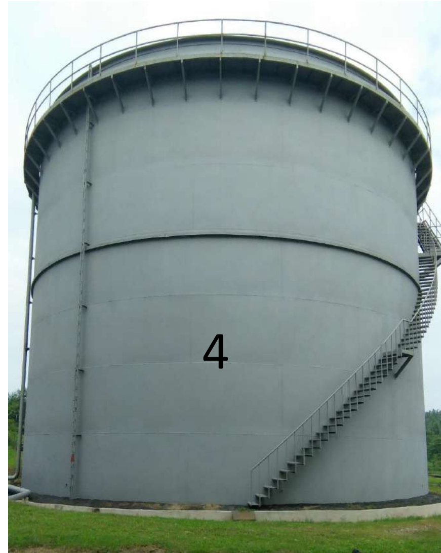
ANAEROBIC DIGESTER NO.4
