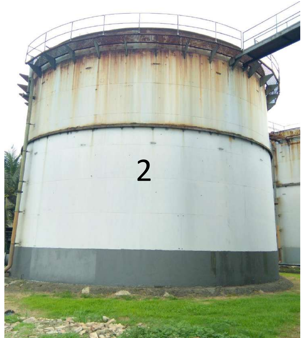
ANAEROBIC DIGESTER NO.2
