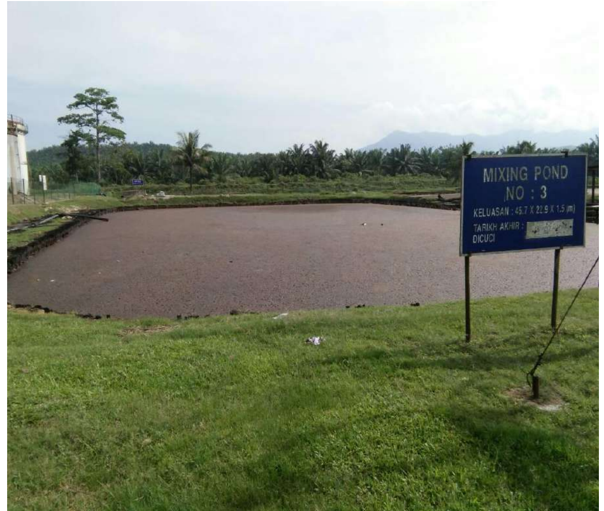
MIXING POND NO. 3
