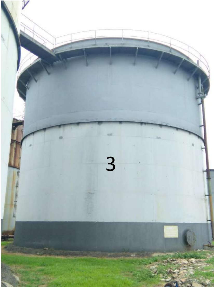
ANAEROBIC DIGESTER NO.3
