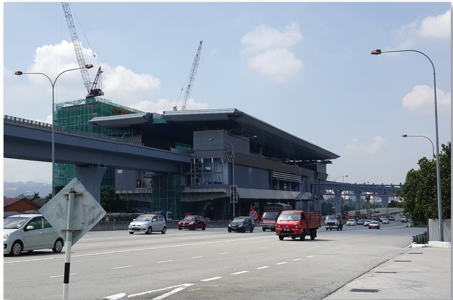
Cheras MRT station in construction phase
