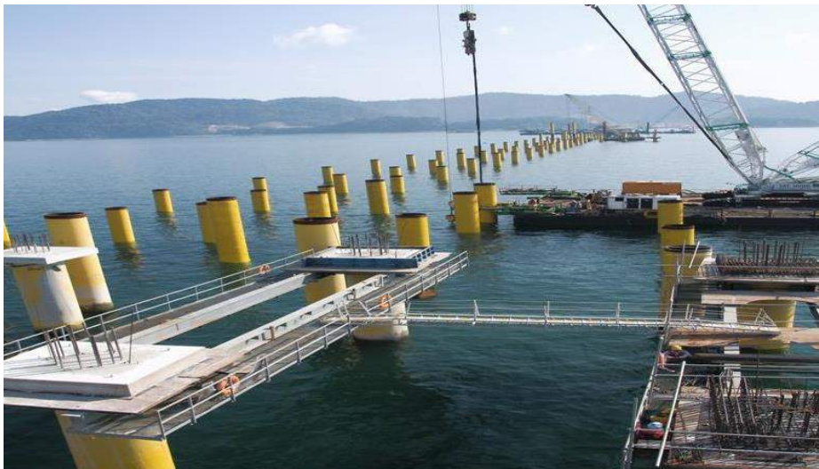
Figure 5.3.1c: Construction of Wharf at Vale, Lumut (Source: http://site.sys.com.my/main/3175/index.asp?pageid=165450&t=Vale%20Main%20Jetty )
