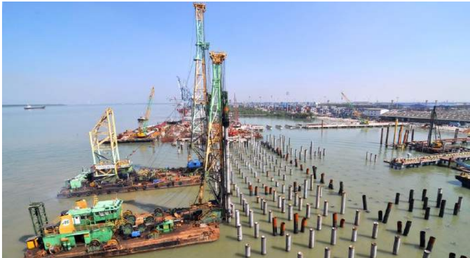
Figure 5.3.1b: Piling Works for Wharf Construction at Northport, Port Klang (Source: http://www.timelapse.com.my/projects/ports-and-marine/ )
