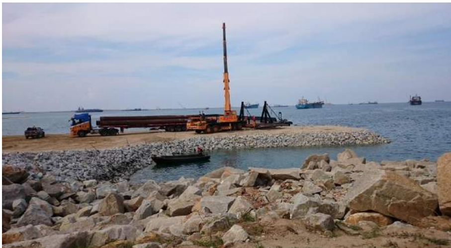
Figure 5.3.1e: Temporary Jetty during Construction at Kuantan Port (Source: G&P)
