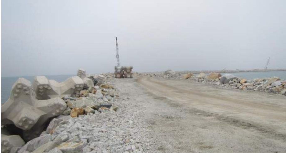
Figure 5.3.1a: Construction of Breakwater at Kuantan Port (Source: G&P)
