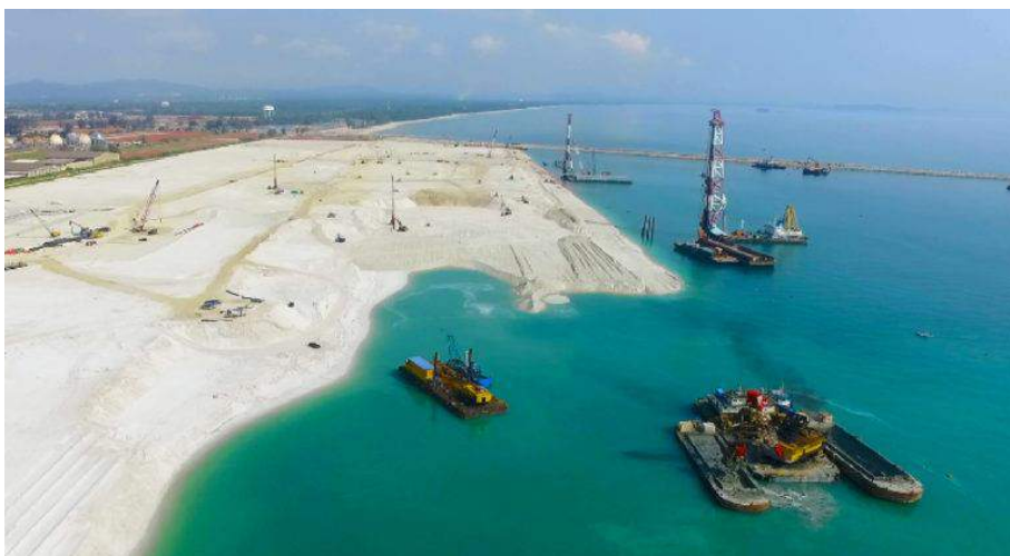
Figure 5.3.1f: Reclamation for Port Development at Kuantan Port (Source: http://www.timelapse.com.my/projects/ports-and-marine/ )
