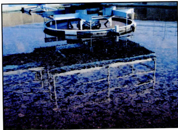
Figure 4.4 Small ash-like particles on surface of clarifier (Source : www.ecoworld.com.vn )
