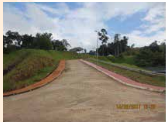
Kawalan Perlindungan Cerun ( Close turfing )
