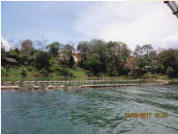
Kawalan Pencemaran Air Larian Permukaan ( Double Silt curtain )
