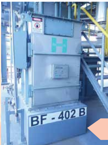
Alat Penapis Bag Udara (Collecting Dust Bag Filter)
