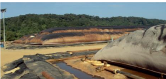
Active Treatment System (ATS)
