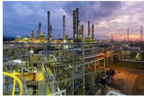
Gas Processing Plant
