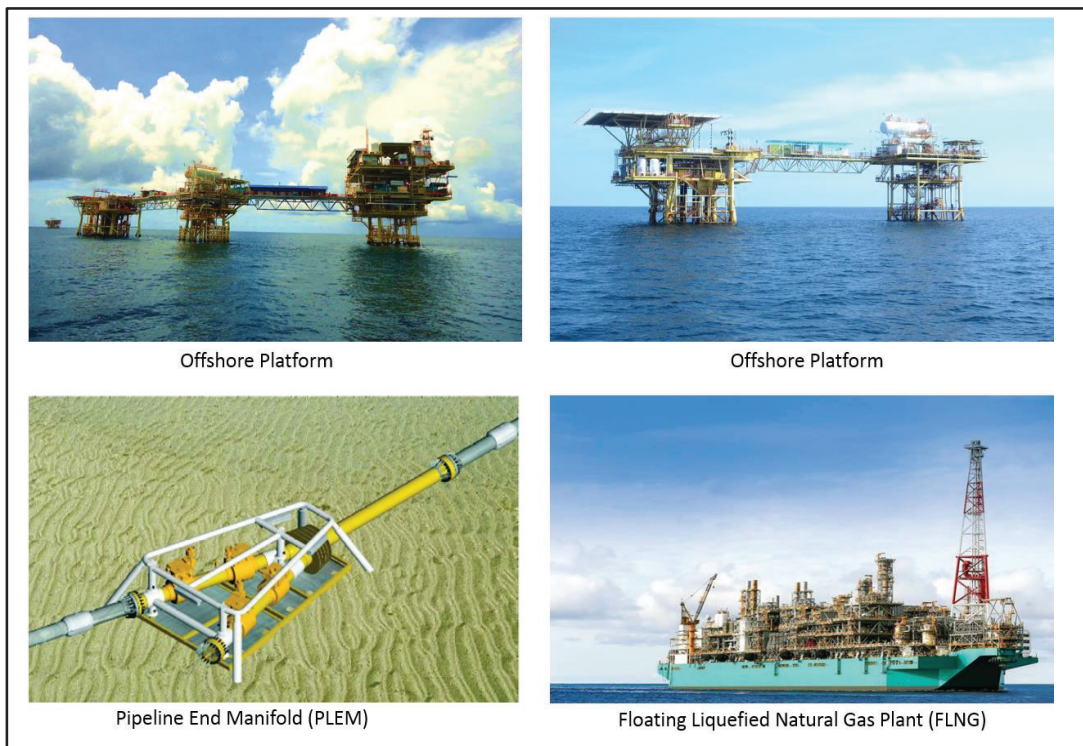
Figure 1.5 Typical Offshore Facilities
