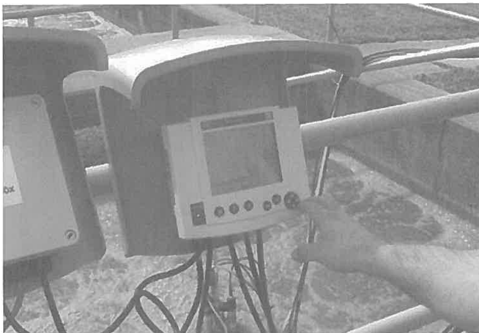
Fig. 17.4: Online ammonia, nitrite, and nitrate monitoring
