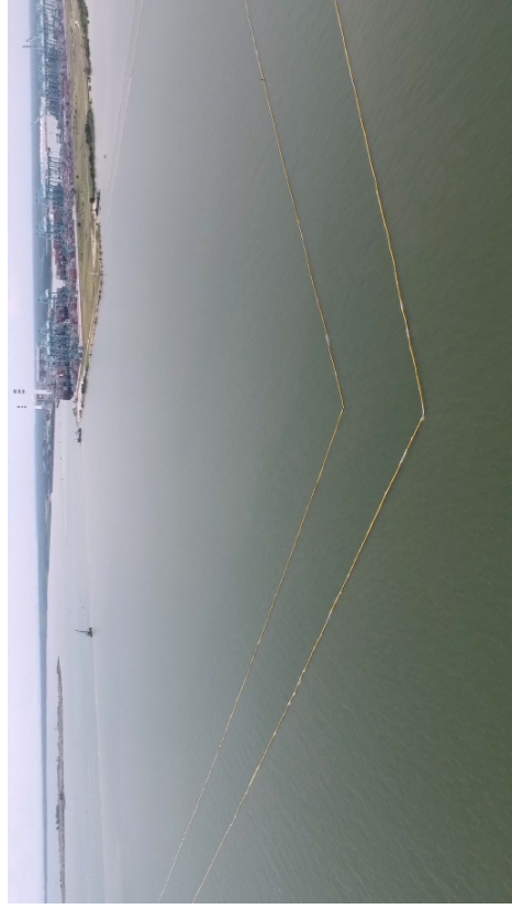
Figure 5.3.1e: Double Layer Silt Curtain
