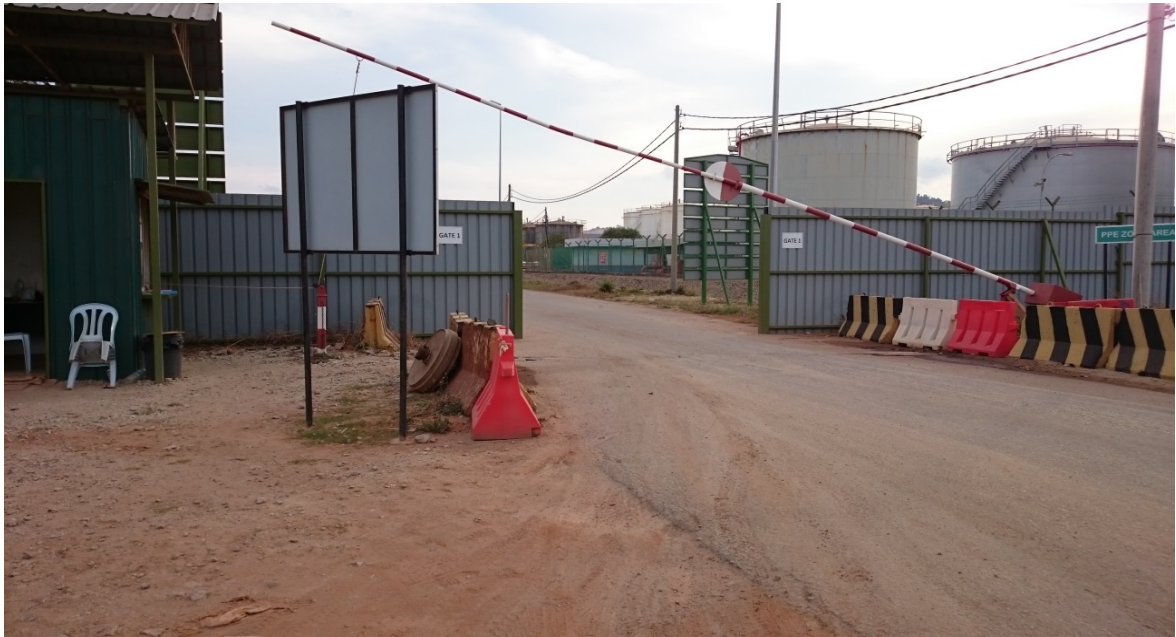
Figure 6.3.2: Example of Site Access and Hoarding
