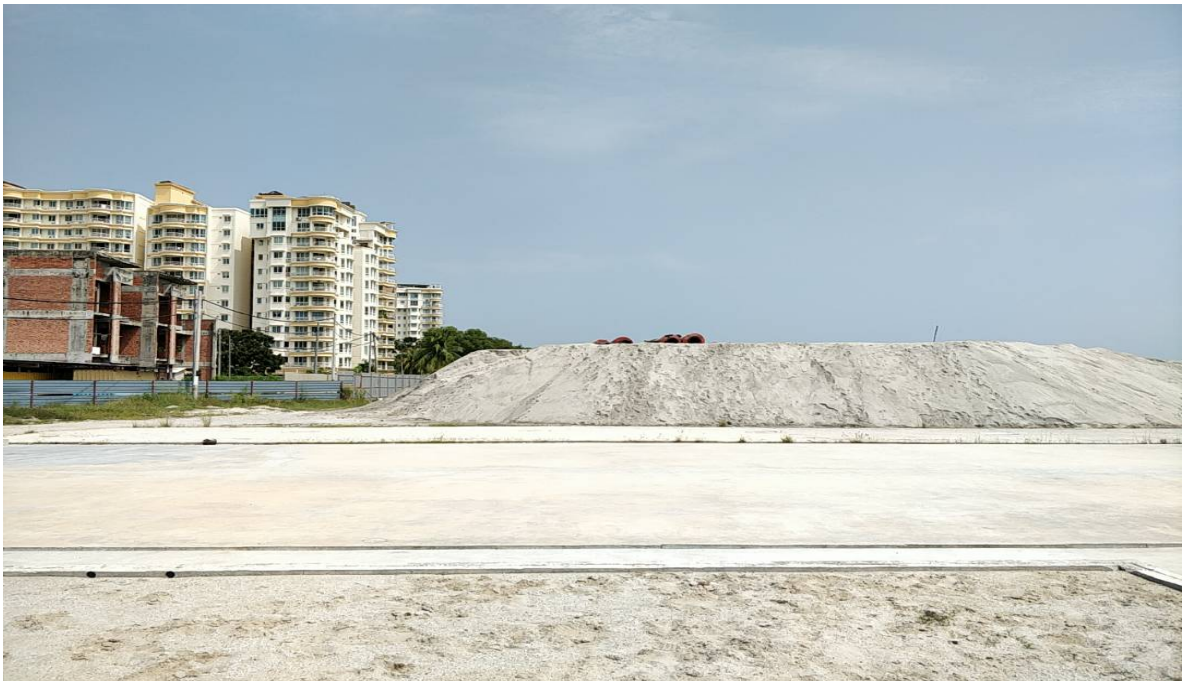
Figure 6.3.13: Surcharge of Land Reclamation Area
