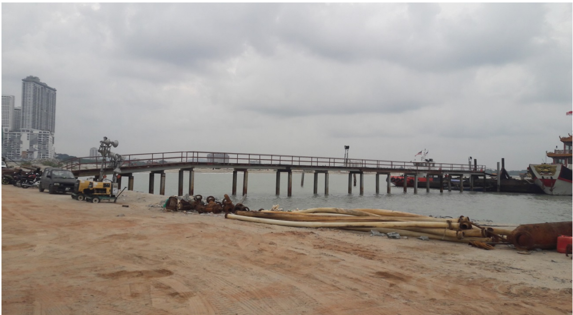
Figure 6.3.3: Example of Temporary Jetty for Land Reclamation Works
