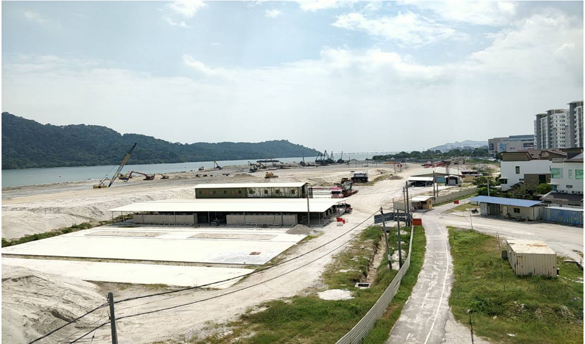
Figure 6.3.4: Example of Site Office and Workers Base Camp
