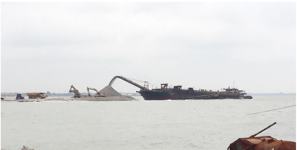
Figure 6.3.8: Sand Filling Works using Conveyor Belt from TSHD
