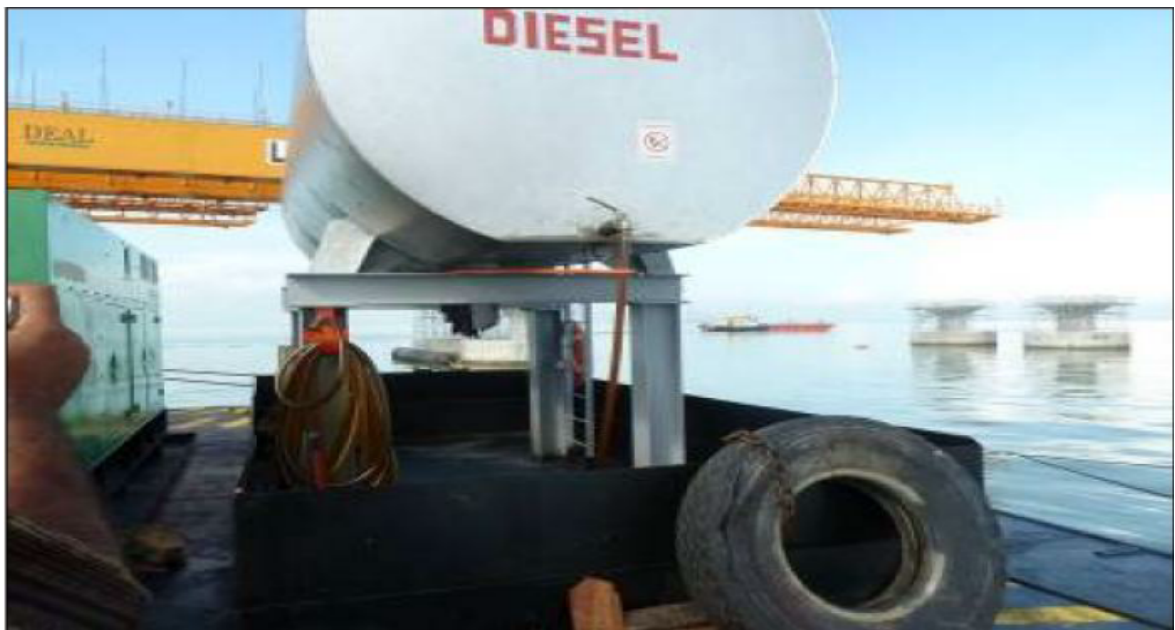
Figure 6.3.5: Example of Skid Tank with Containment Tray
