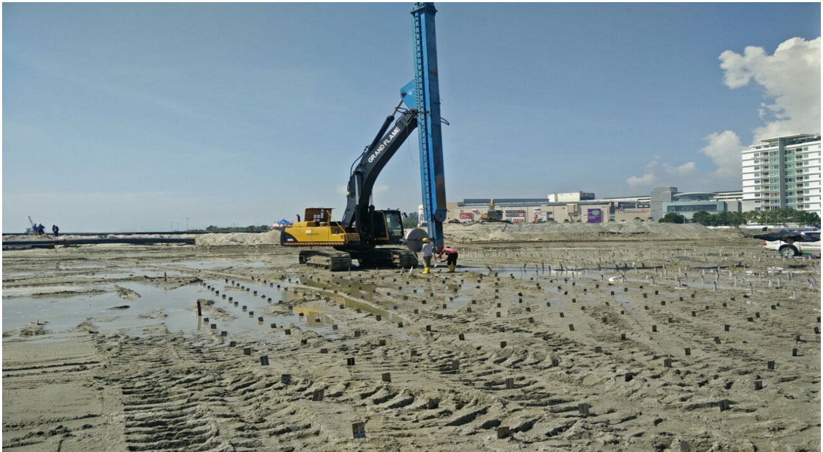
Figure 6.3.11: Ground Treatment Works using PVD System
