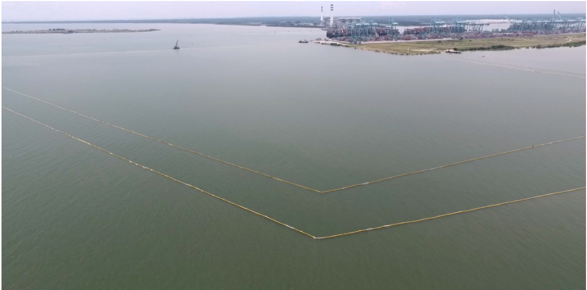
Figure 6.3.7: Example of Installed Silt Curtain prior to Land Reclamation Works
