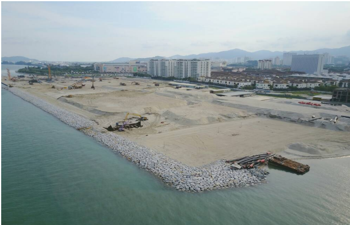
Figure 6.3.14: Example of Rock Revetment Construction Works
