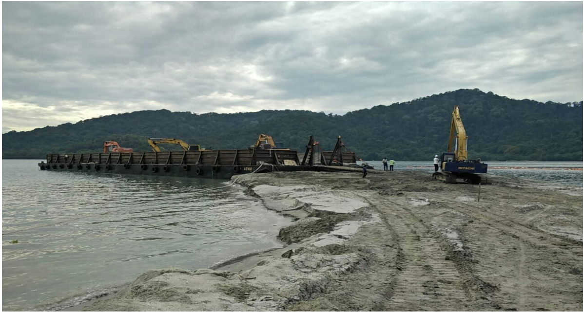
Figure 6.3.9: Construction of Sand Containment Bund using Flat Top Barge and Excavator
