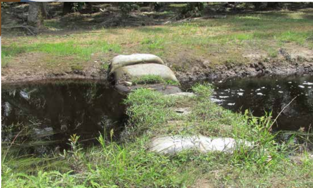
Gambar 4.11 : Check Dam Geobag
