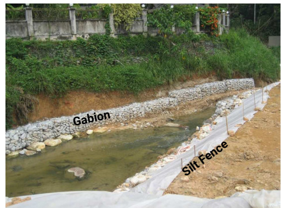
Slit Fence and Gabion
