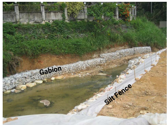
Silt Fence and Gabion
