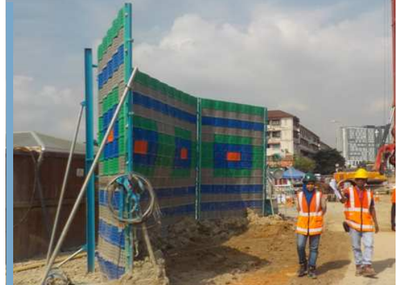
Temporary Noise Barrier
