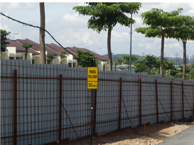
Speed Limit Signage
