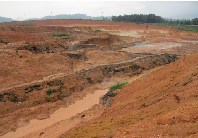
Soil erosion on worked slope
