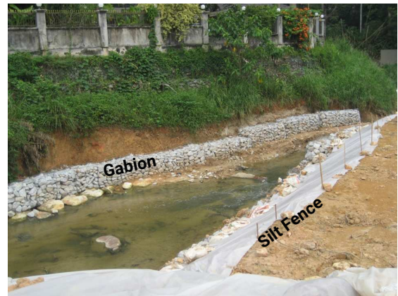
Silt Fence and Gabion
