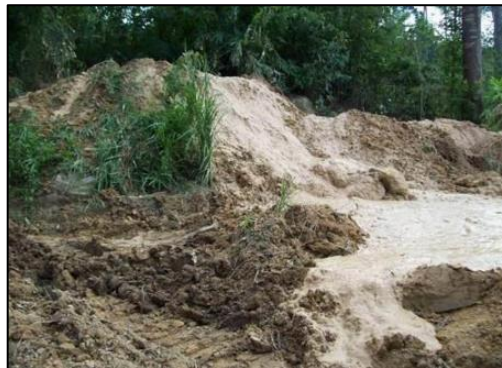
Improper management of spoils
