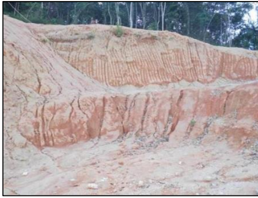
Soil erosion from worked slopes
