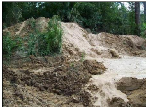
Improper management of spoils
