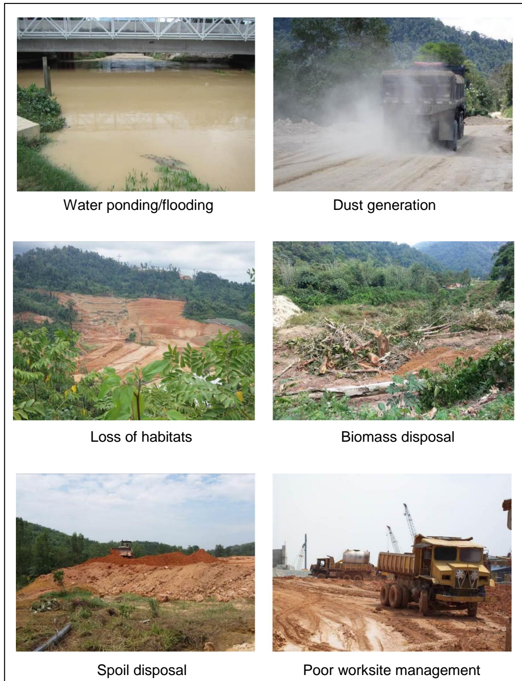
Figure 5.1(b): Photo Inventory of Common Impacts associated with Chemical Plants Development
