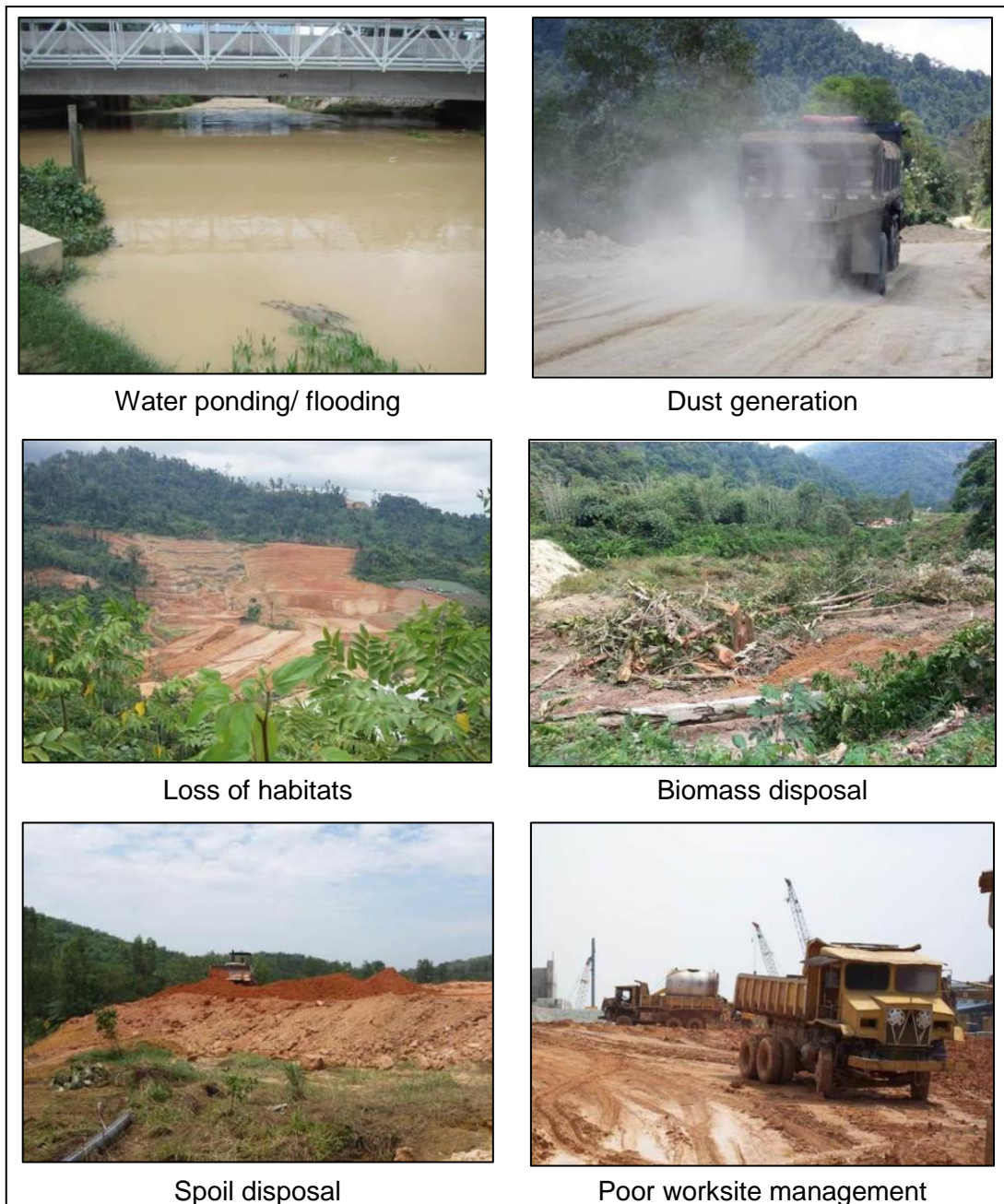
Figure 5.3 (b): Photo Inventory of Common Impacts associated with Shipyard Development
