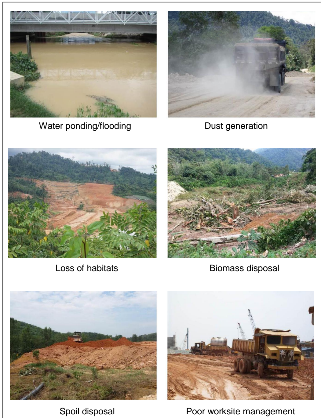
Figure 5.1(b): Photo Inventory of Common Impacts associated with Non-ferrous Manufacturing Plants Development
