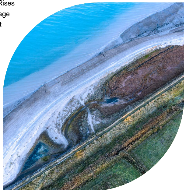
Coastal defences on the River Orwell Suffolk, United Kingdom, a traditional sea wall and a "nature like" constructed mudflat that not only protects the sea wall but also provides wildlife habitat.
