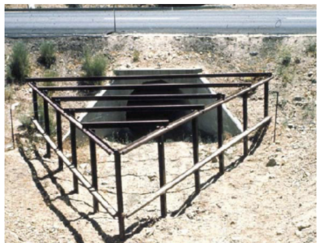
Figure 15. Upstream view of a steel debris deflector
