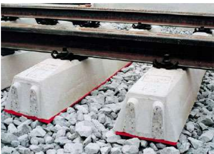
Plate E-23: Under sleeper pads vibration isolation of railway tracks
