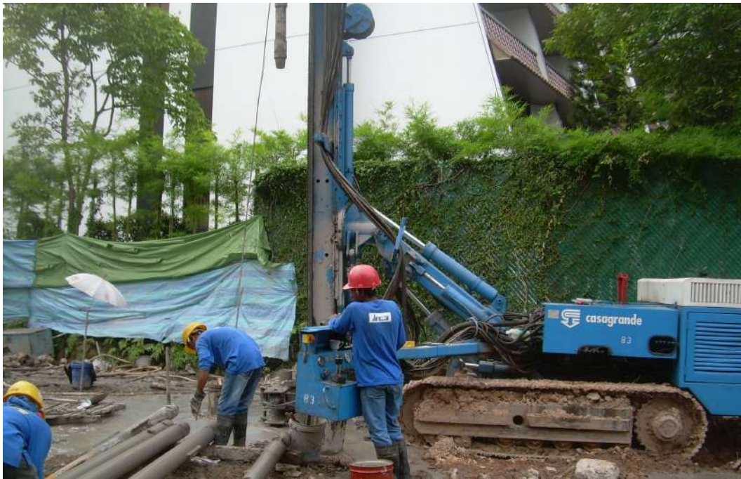
Plate E-12: Example of bored micro-piling in a work site adjacent residential receptor
