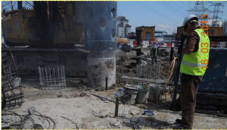
Plate C-1: Vibration testing of pile driving in MRT work site for piling vibration predictions
