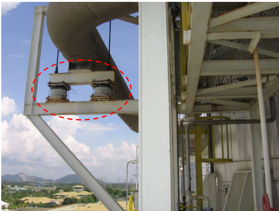
Plate E-28: Vibration isolator and viscous dampers installed in industrial facilities
