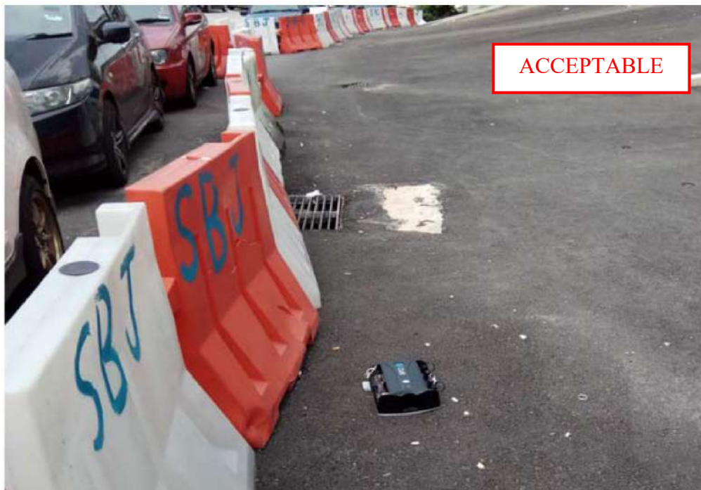
Plate B-26: Use of integrated vibration monitoring equipment placed onto road surface avoid problems of rigid coupling of geophone sensor type monitoring equipment
