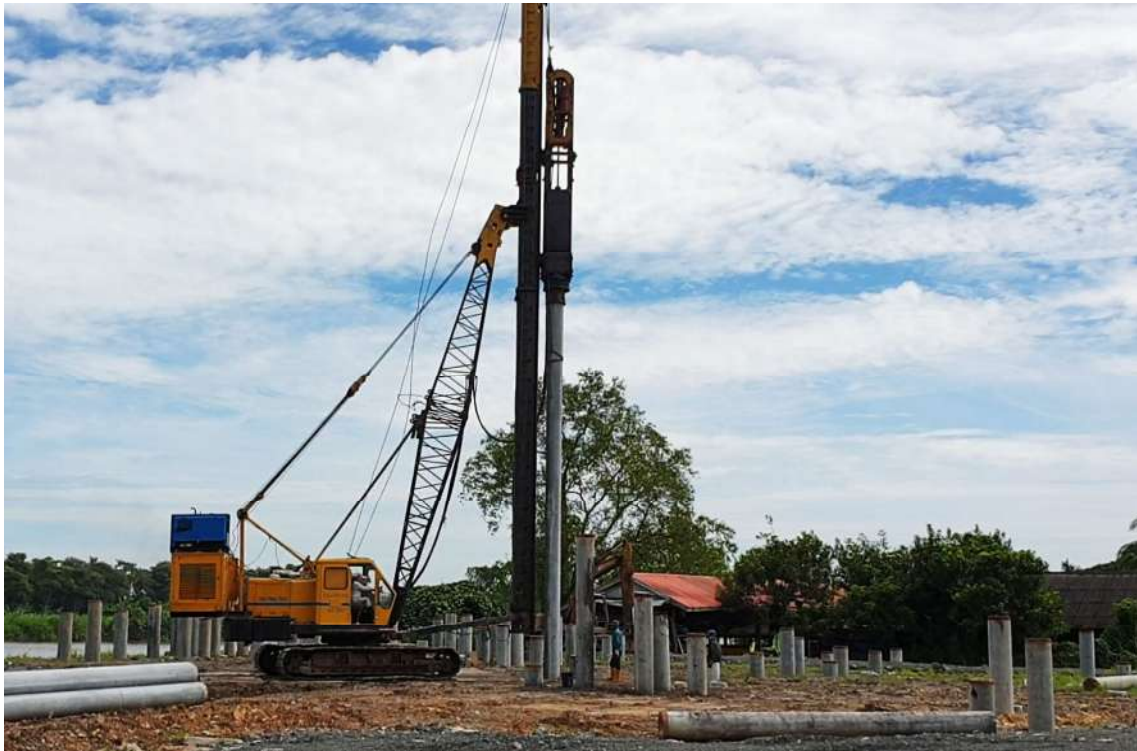
Plate E-2: Example of hammer driven piling in progress (Kuching, Sarawak)
