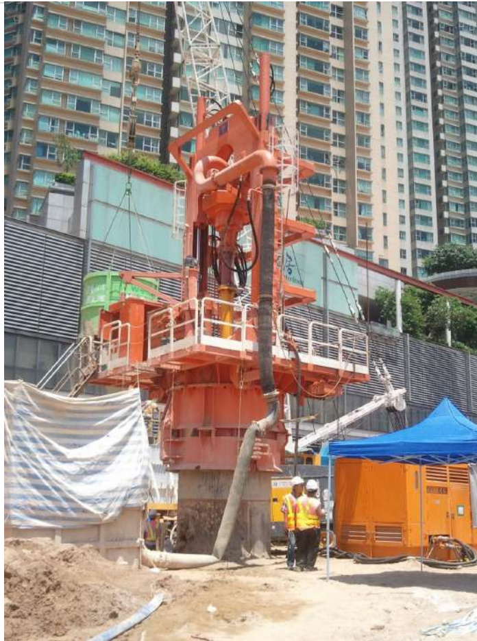
Plate E-6: Reversed circulation drilling in an urban underground train station work site (Kowloon, Hong Kong)
