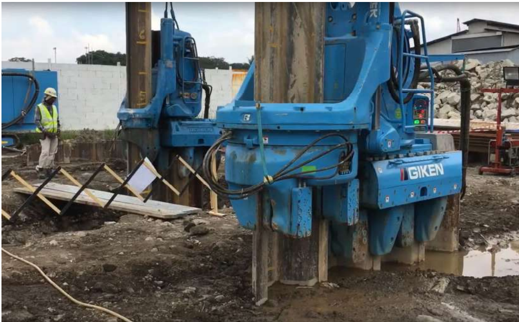
Plate E-8: Pressed-in sheet piling using proprietary silent piler in urban work site
