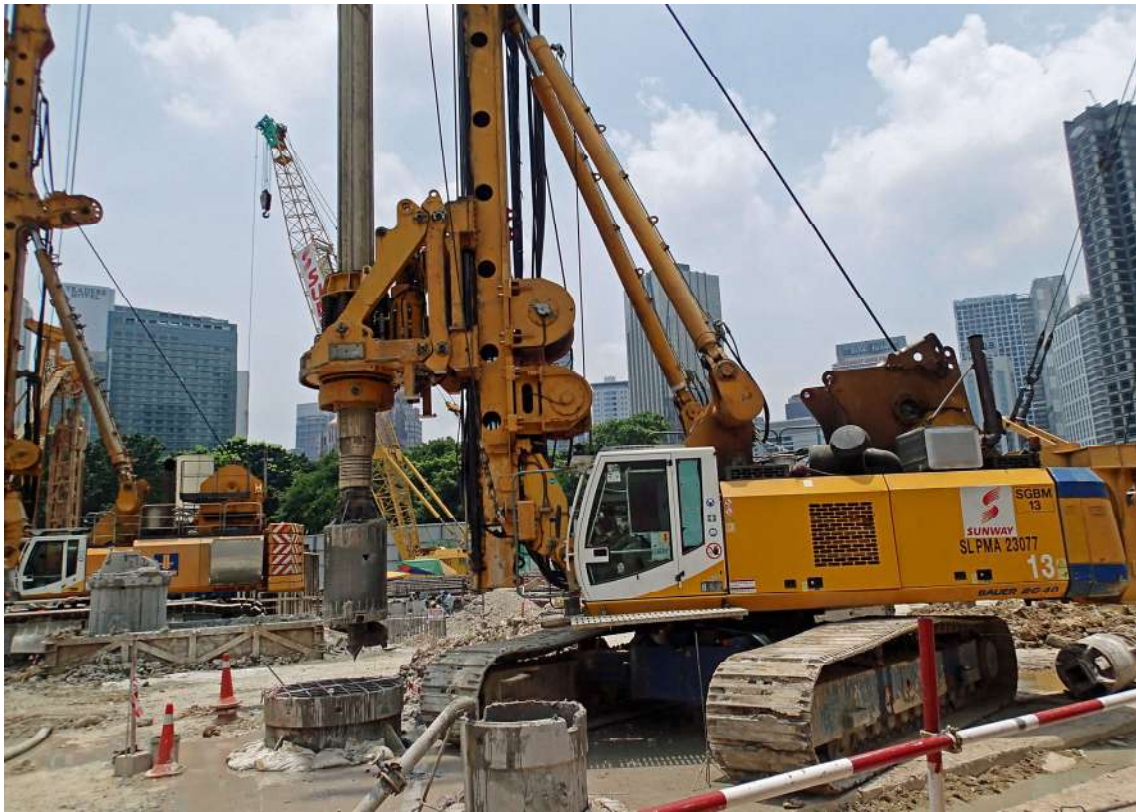
Plate E-4: Rotary bored piling in an urban project site (KLCC Kuala Lumpur)
