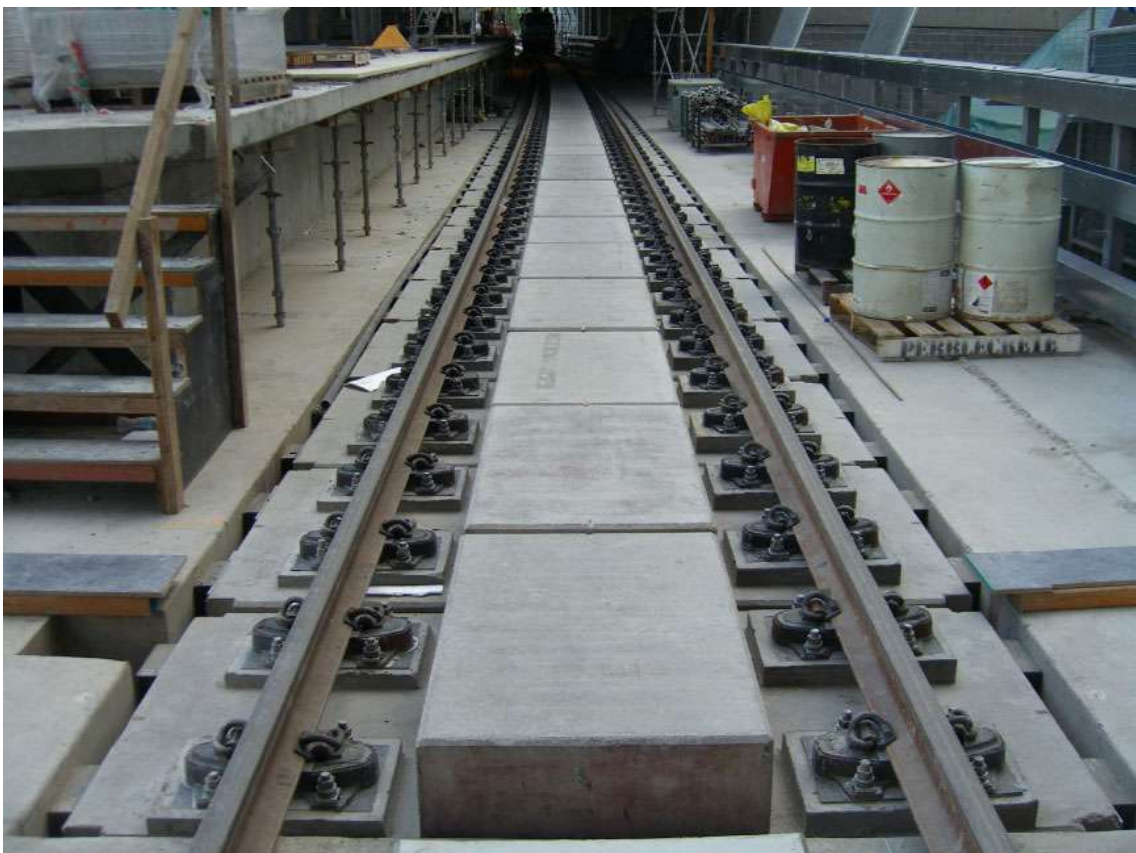
Plate E-27: Newly completed floating slab track (Chatswoods Station, Sydney)
