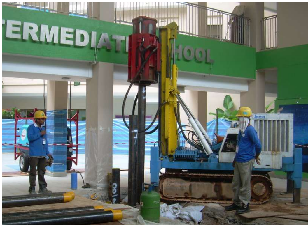
Plate E-13: Example of driven micro-piling in a congested sensitive work site
