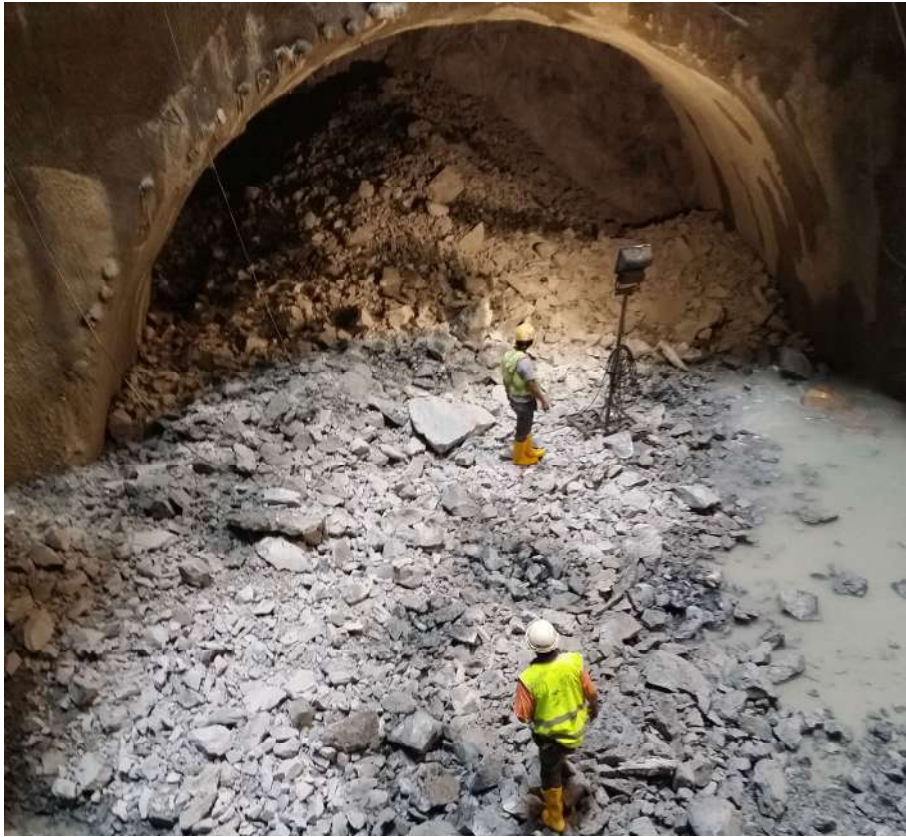
Plate E-14: Optimal explosives (charge per delay) and rock removal in tunneling for blast induced vibration mitigation in tunneling project (NS2 Tunnel Singapore)
