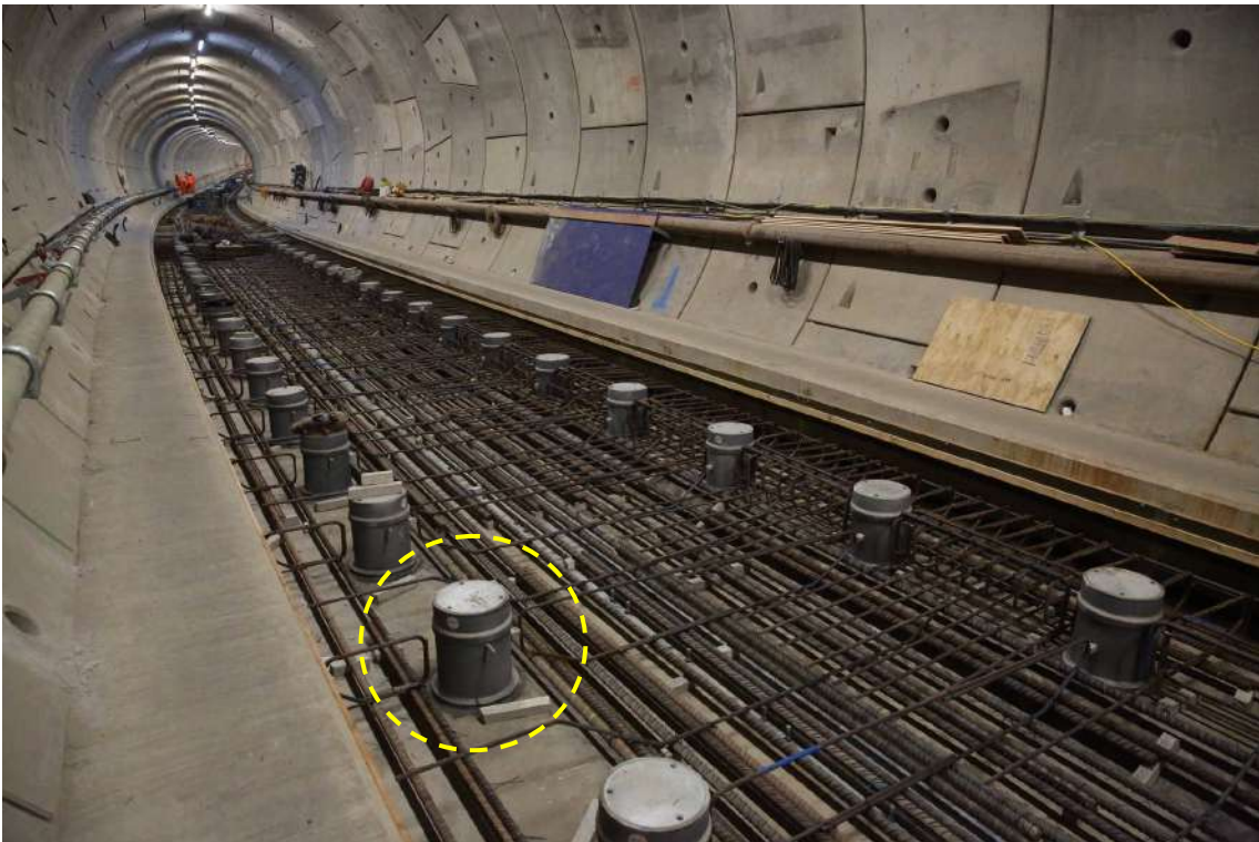
Plate E-26: Floating slab track using discrete isolation mounts - under construction with rebars and vibration isolators installed awaiting concrete pour (Crossrail, United Kingdom)
