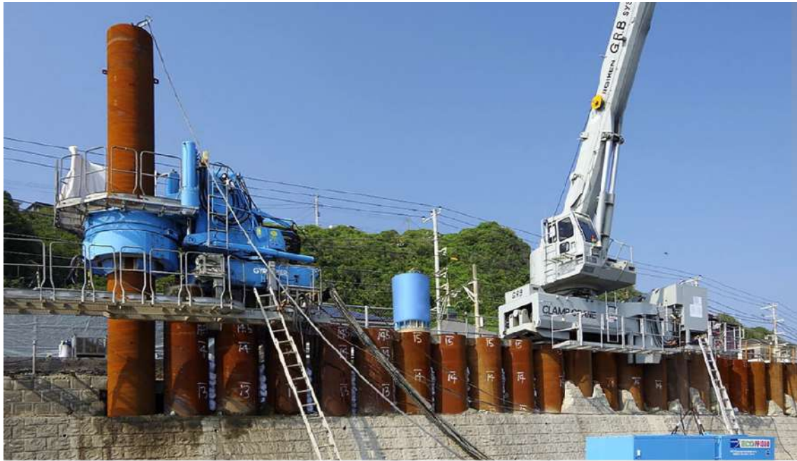
Plate E-10: Example of retaining wall construction using gyro press press-in piling method
