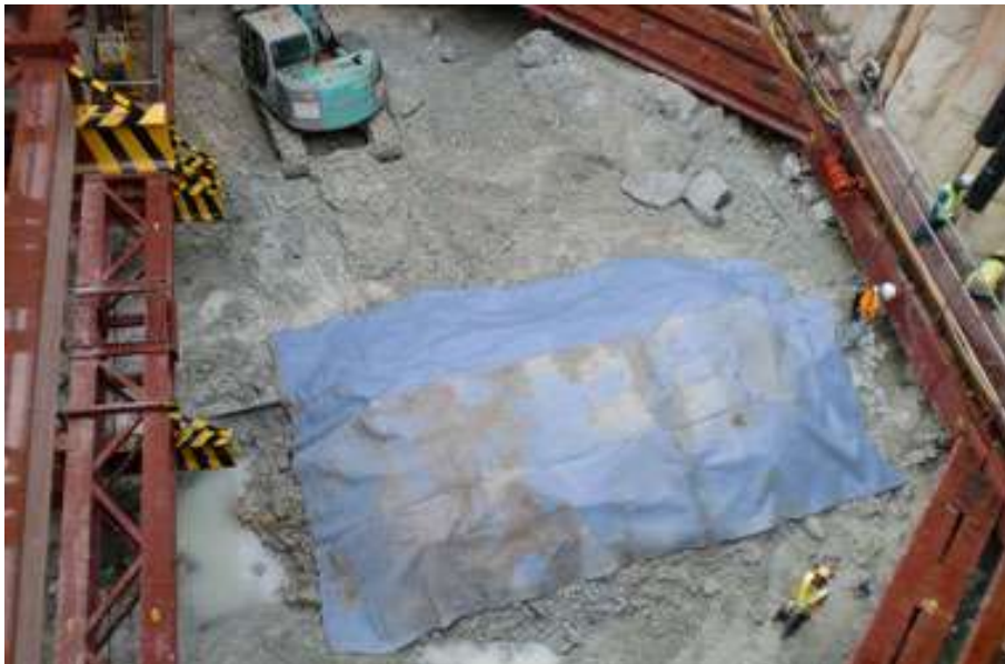
Plate E-15: Controlled blasting in an urban condominium construction project (Singapore)
