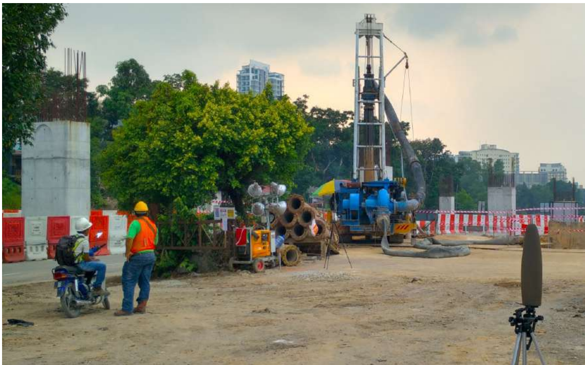
Plate E-6: Reversed circulation drilling in an urban underground train station work site (Kowloon, Hong Kong)
