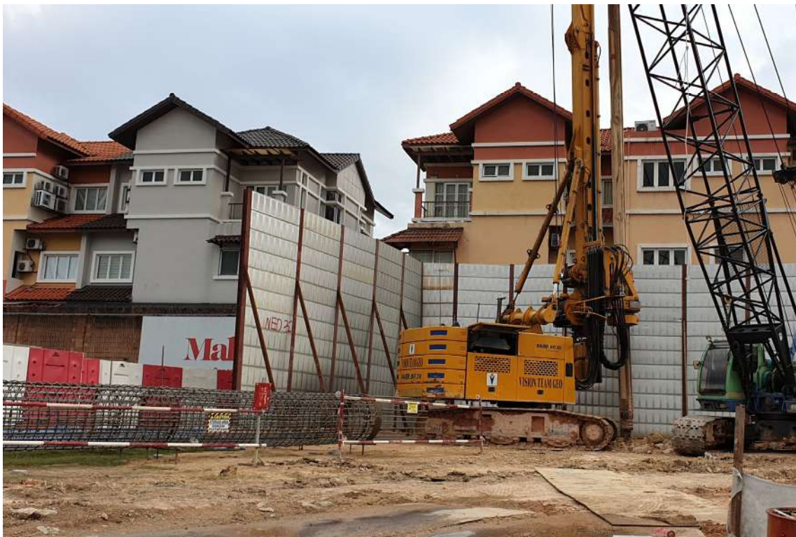
Plate E-5: Rotary bored piling in an urban transit rail project adjacent residential receptor (Klang Valley LRT3, Petaling Jaya)
