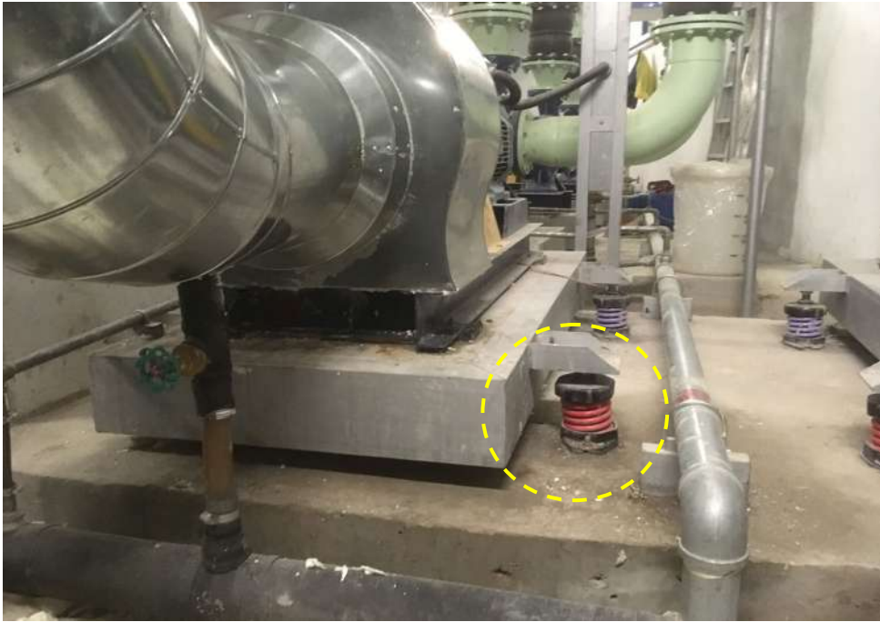
Plate E-30: Example of vibration isolators for generators
