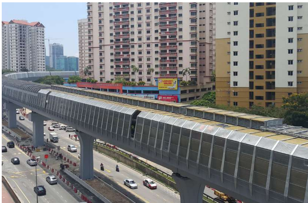
Figure E-16: Full enclosure for MRT trains noise mitigation adjacent sensitive receptors in high rise buildings
