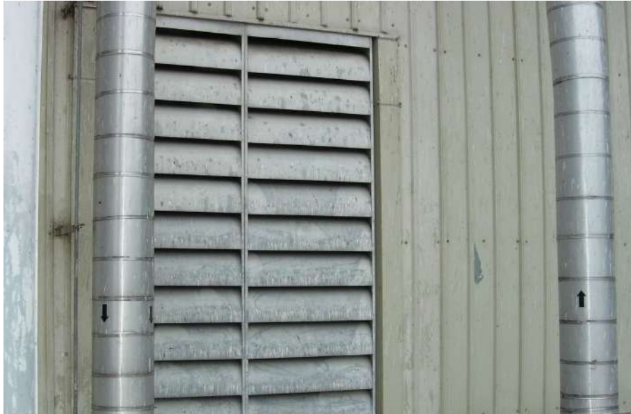
Figure E-22: Acoustic louvers used for natural ventilation opening in power station turbine hall
