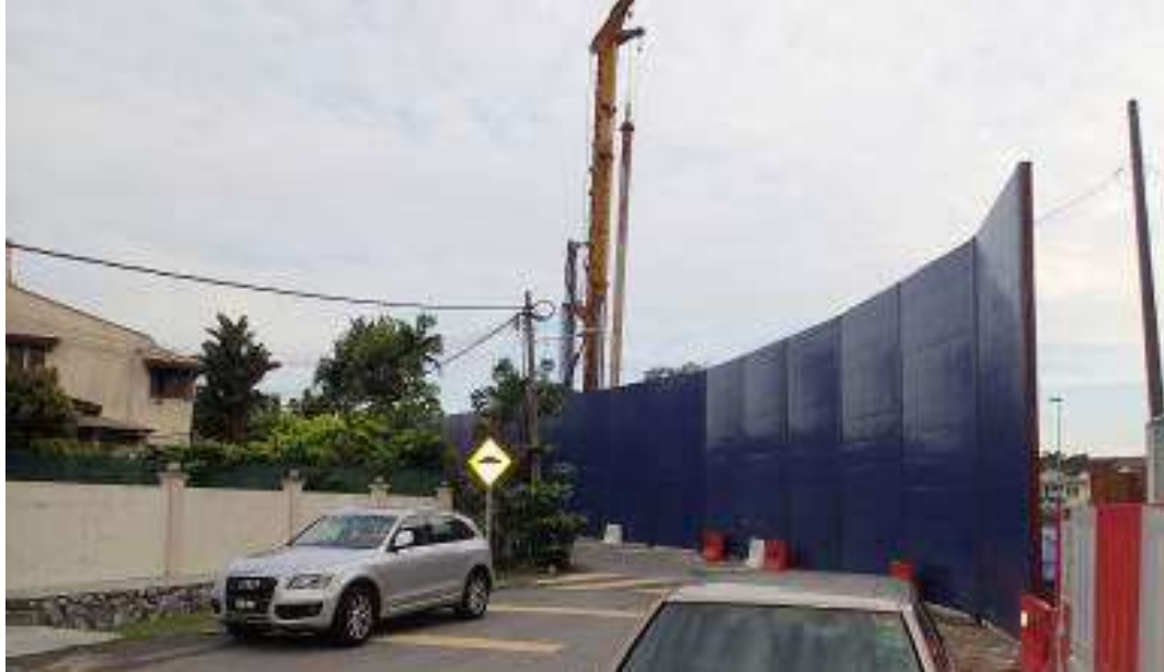
Figure E-9: Temporary noise barriers used in construction noise mitigation
