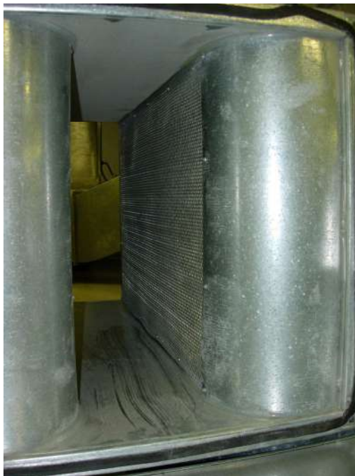
Figure E-20: Dissipative silencers in a plantroom application, with a close up view of typical sound absorption splitters
