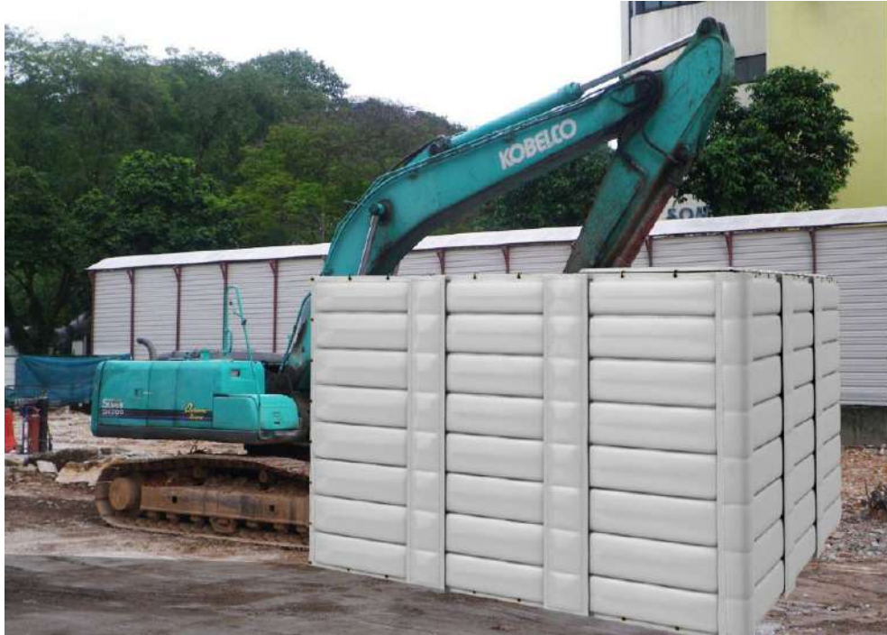
Figure E-11: Movable barriers used for mobile noise source in construction works
