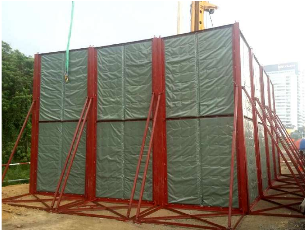
Figure E-12: Movable barrier used for piling noise mitigation
