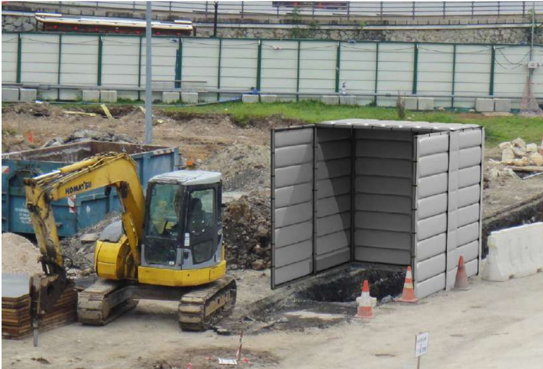
Figure E-18: Movable partial enclosures for construction works noise mitigation
