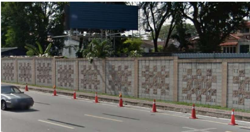
Figure E-8: Masonry noise barriers used in highway noise mitigation
