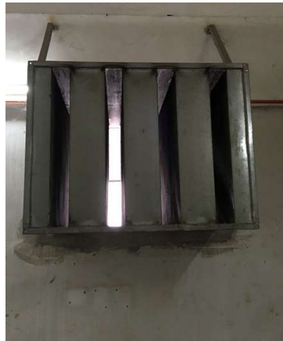
Figure E-20: Dissipative silencers in a plantroom application, with a close up view of typical sound absorption splitters
