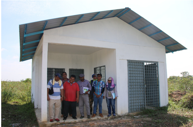
Gambar 33: Rumah pam air, Hutan Simpan Raja Musa, Kuala Selangor, Selangor
