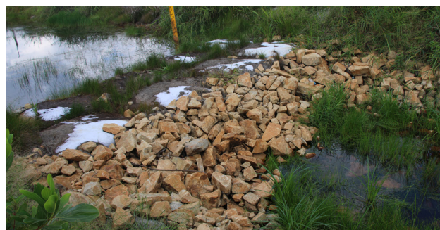
Gambar 9: Sekatan saluran "geobag and rocks", TCD 3, Sungai Bukit Takal, Kemaman, Terengganu
