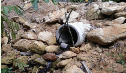
ii. PAM Block Polymer at culvert
