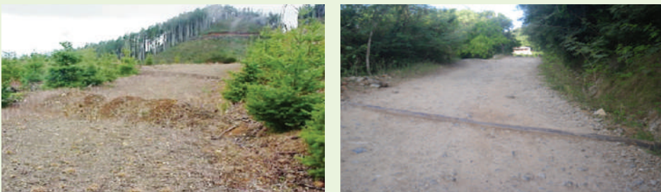
Water Bar crossing the access road.
