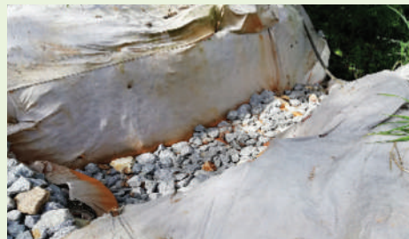
ii. Riprap installation inside the discharged outlet
