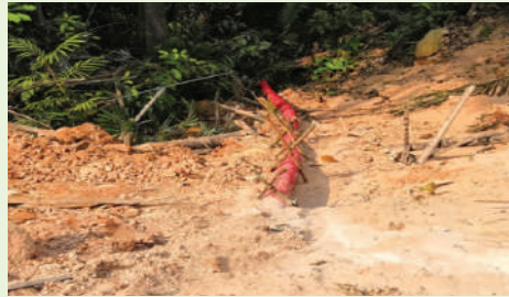
iii. Slope drain pipe
