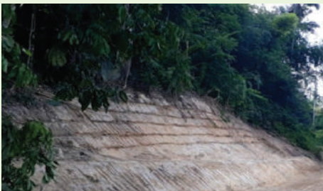
i. Horizontal groove before hydroseeding
