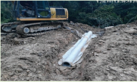
i. Installation of culvert crossing in progress
