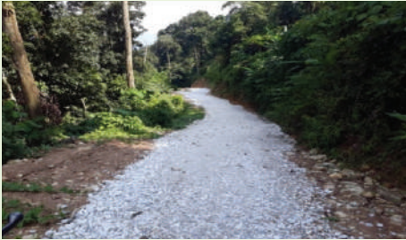
i. Gravel at access road
