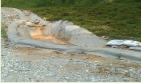
i. Sandbag covered with geotextile sheet around and inlet/outlet of silt trap
