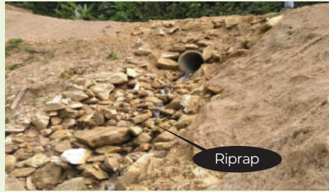
iv. Culvert installation
