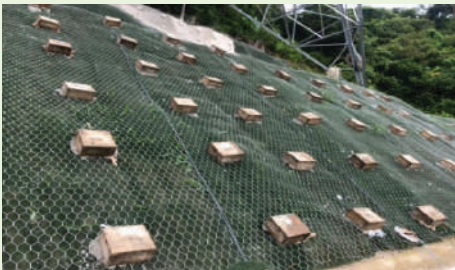
iii. Steel Grid Netting with Soil Nail Head
