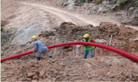
i. Installation of slope drain pipe using corrugated plastic pipe
