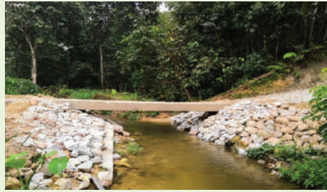
i. Bridge installation for river crossing
