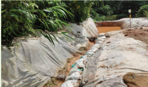
i. PAM Block Polymer at sediment basin
