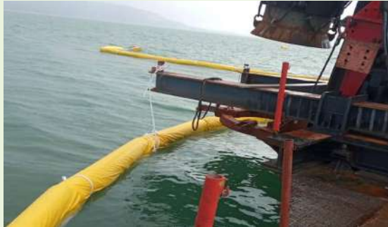
Example of silt curtain installation.
