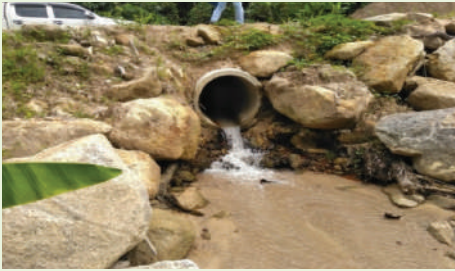
iii. Culvert installation
