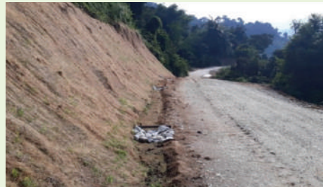
ii. Check dam installation along the earthdrain
