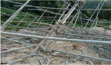
iii. Steel Grid Netting with Soil Nail Head
