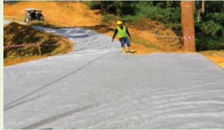
ii. Gravel installation at waterways crossing required geotextile sheet
