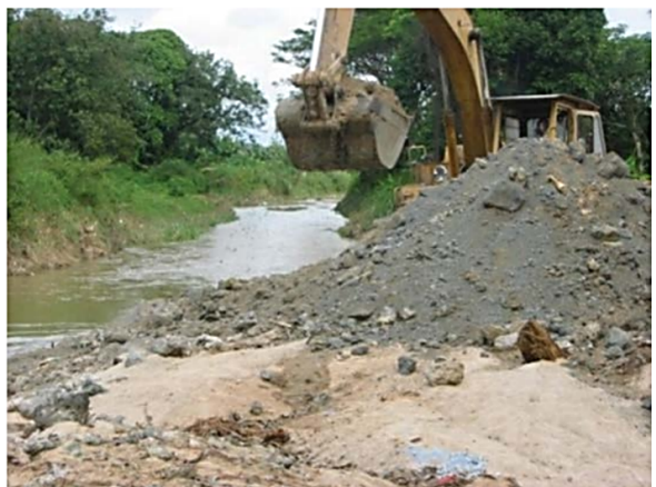
Fig. 1. Removing wastewater sludge from the river [15].
