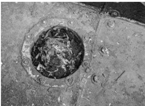
Figure 9.43 Blocked outlets — materials may vary from screw caps to leaves (Heriot-Watt University)
