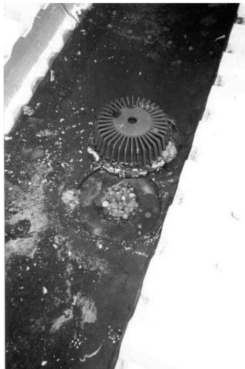
Figure 9.43 Blocked outlets — materials may vary from screw caps to leaves (Heriot-Watt University)
