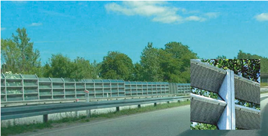
[67] Copenhagen, Denmark Steel and glass barrier
