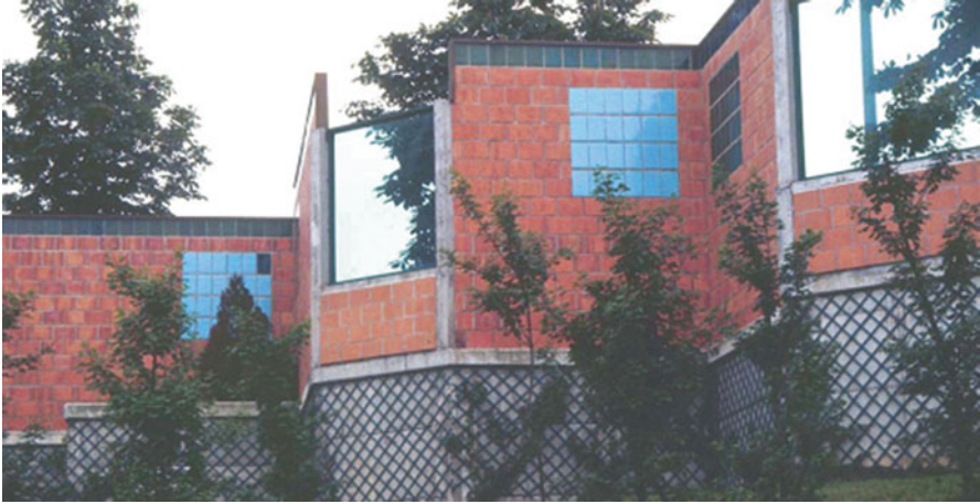
[67] Paris, France Glass and brick noise barrier
