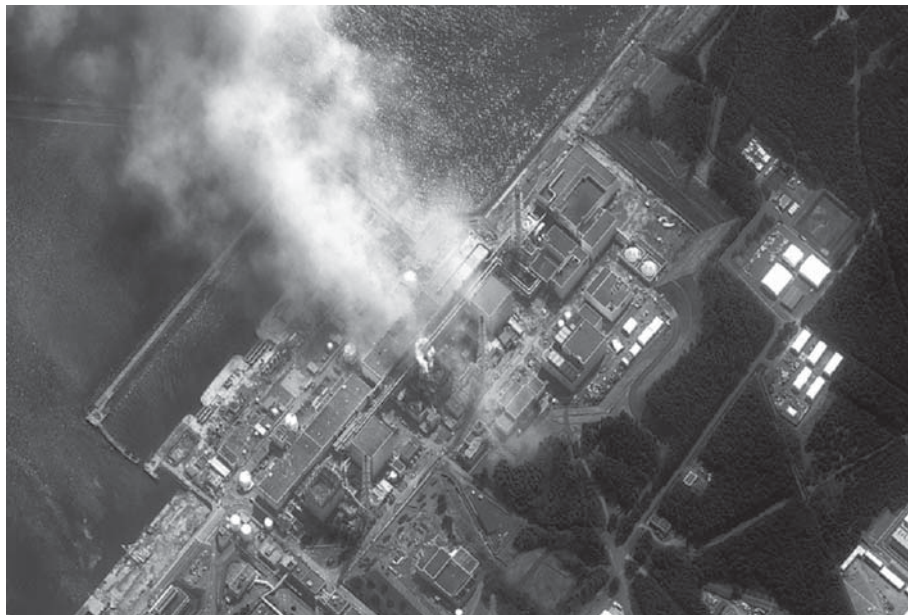
FIGURE 1.5 Aerial view of release at nuclear reactors at Daiichi plant, Fukushima, Japan. (From asianews.it.)
