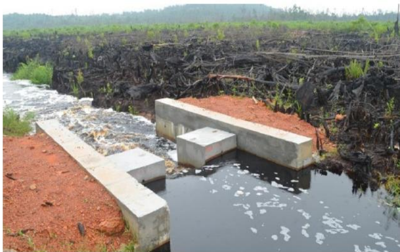
Gambar 4.10: Check Dam Konkrit
