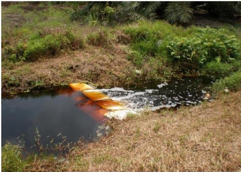
Gambar 4.9: Check Dam Geobag
