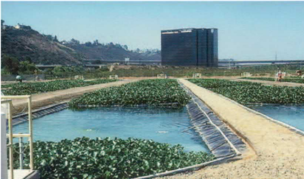
FIG. 31.11 Engineered and constructed wetland system in San Diego, California, utilizing macrophytes, that is, water hyacinths ( Eichhornia spp.). The system takes advantage of both microbial and larger plant species (bioremediation and phytoremediation, respectively). Source: C.P. Gerba, I.L. Pepper, Wastewater treatment and biosolids reuse , in: Environmental Microbiology , second ed., Elsevier Inc., USA, 2009, pp. 503–530.
