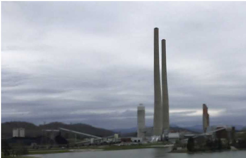
FIG. 7.1 Kingston steam electric generating station on the Emory River, Tennessee. This 1.4-gigawatt coal-fired power plant is located next to Watts Bar Lake and is operated by the Tennessee Valley Authority. The plant is the site of a large fly ash spill in December 2008. Courtesy of D.A. Vallero.
