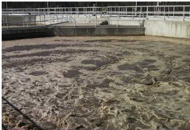
FIG. 31.9 Aerobic treatment approach to degrade hazardous waste. In this activated sludge treatment system, the waste is combined with recycled biomass and aerated to maintain a target dissolved oxygen (DO) content. Organisms use the organic components, expressed as biochemical oxygen demand (BOD) of waste as food, decreasing the organic levels in the wastewater. Oxygen concentrations must be controlled to maintain optimal treatment efficiencies. One means of achieving optimal DO content is tapered aeration, which provides highest concentrations of oxygen near the influent to accommodate the large oxygen demand from microbes as waste is introduced to the aeration tank (photo). Adapted from D.A. Vallero, J.J. Peirce, Engineering the Risks of Hazardous Wastes , Butterworth-Heinemann, Burlington, MA, 2003, pp. xxi, 306 p.; photo courtesy of D.J. Vallero.
