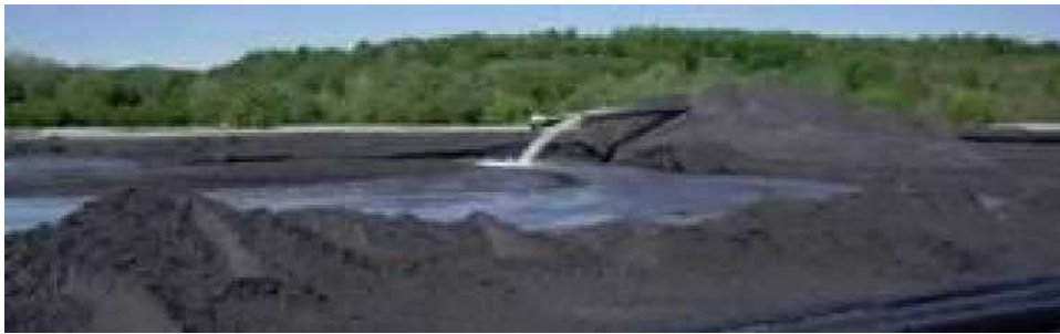
FIG. 7.6 Coal ash staging area. The ash slurry is pumped from the power plant and released into an ash impoundment. Courtesy of U.S. Environmental Protection Agency, Coal Ash (Coal Combustion Residuals, or CCR) , 2018, March 8, 2018. Available from: https://www.epa.gov/coalash .
