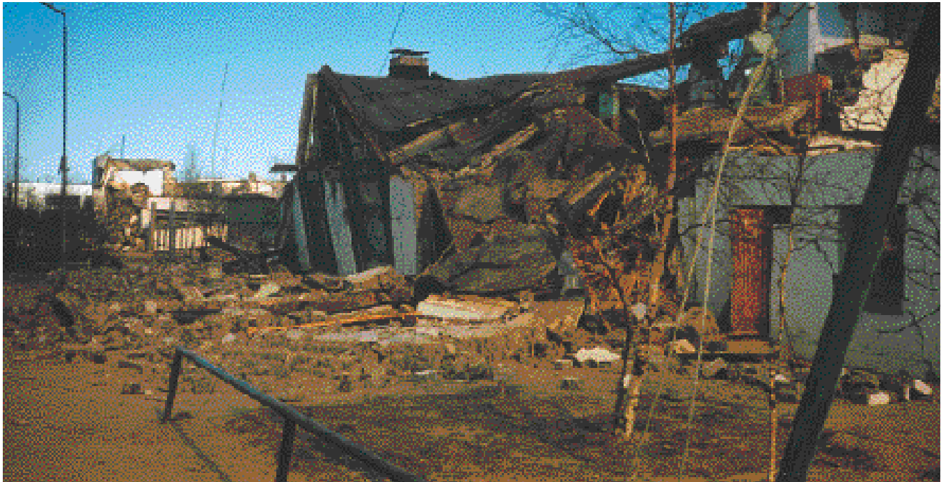
Figure 1: The completely damaged shop building in Neftegorsk
