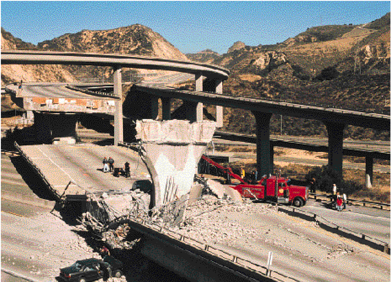
Los Angeles earthquake: Large, elevated sections of the main highway collapsed in 1994
