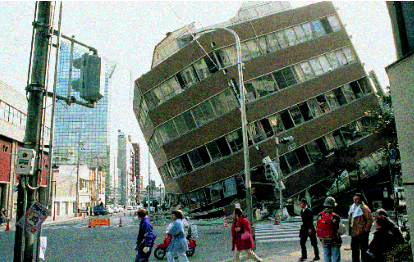
Destruction to property caused by the Kobe earthquake in Japan
