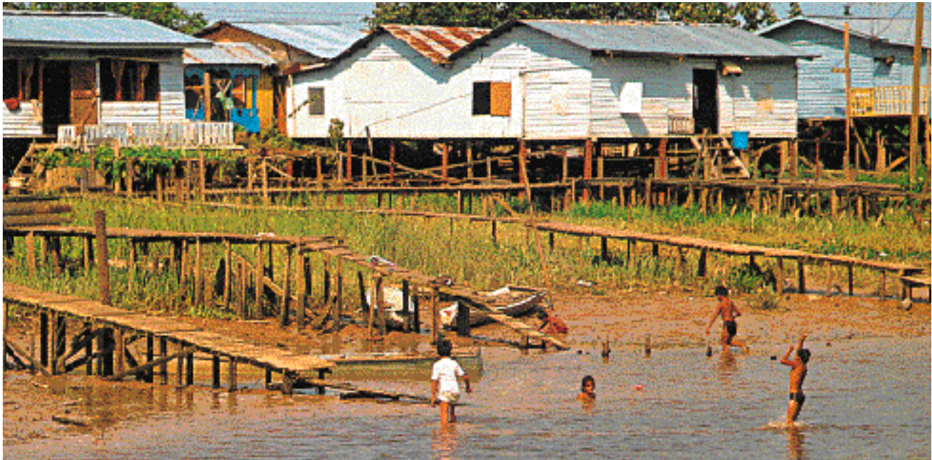
Figure 1: The traditional Malay 'stilt-house' as an effective defence mechanism against flooding. The houses are 'clustered' and joined by wooden walk-ways to further strengthen the houses against strong river currents during flooding
