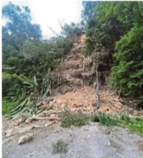
A 30m landslide destroyed part of a slope near the Taman Cheras Mas apartments on Nov 25. PIC COURTESY OF THE FIRE AND RESCUE DEPARTMENT
