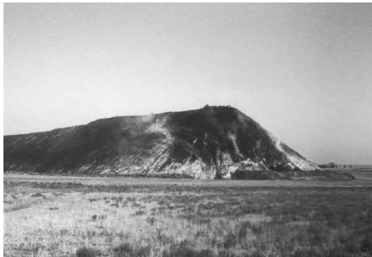
FIG. 6.6 A burning dump of coal waste.
