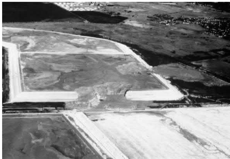
FIG. 6.12 Failures of a gold tailings storage at Saaiplaas mine that was being built at an excessive rate of rise. (Two failures are visible, side by side in the center of the photograph, and one in the center-right.)
