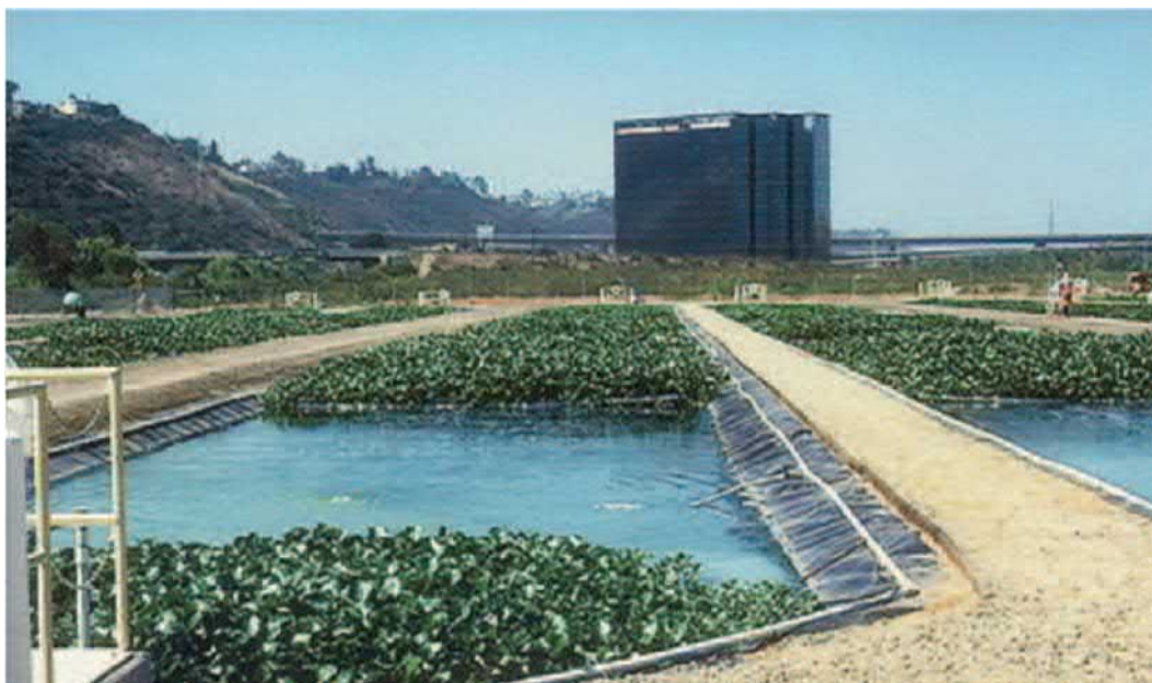
FIG. 31.11 Engineered and constructed wetland system in San Diego, California, utilizing macrophytes, that is, water hyacinths ( Eichhornia spp.). The system takes advantage of both microbial and larger plant species (bioremediation and phytoremediation, respectively). Source: C.P. Gerba, I.L. Pepper, Wastewater treatment and biosolids reuse , in: Environmental Microbiology , second ed., Elsevier Inc., USA, 2009, pp. 503–530.
