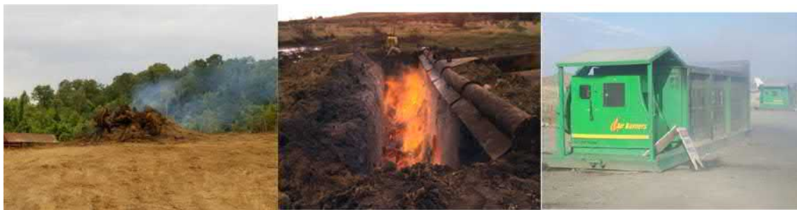
FIG. 29.4 Incineration of vegetative material. The left of open pile burning. The middle is a trenched air curtain and the right is a containerized air curtain system.
