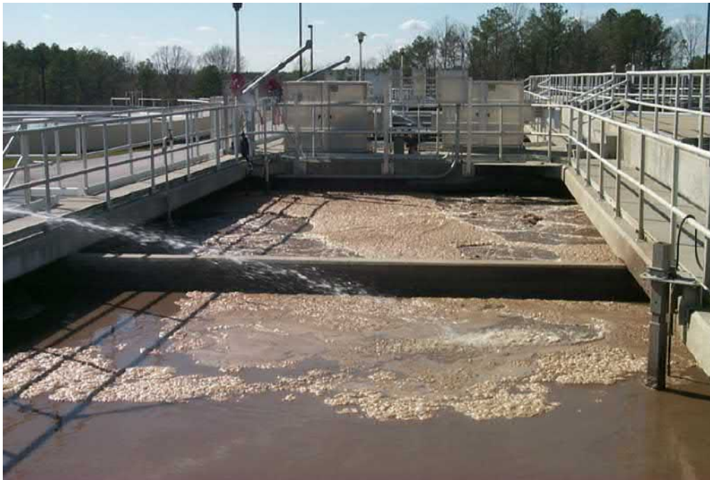
FIG. 31.13 Anaerobic treatment system. The lighter substances have migrated to the surface. These may be fats that have been separated physically during the treatment process, or bubbles from gases, such as methane, that are produced when the anaerobes degrade the wastes. Note that although this is an anoxic chamber, a thin film layer at the surface will be aerobic because it is in contact with the atmosphere. Photo courtesy of D.J. Vallero.
