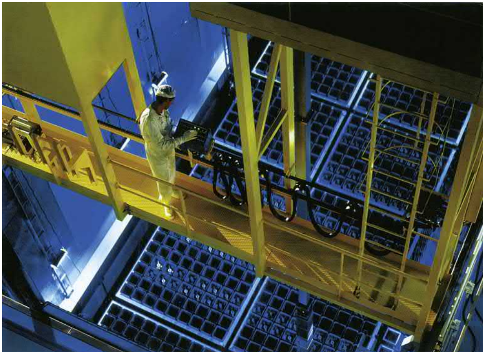
FIG. 11.1 Typical cooling basin for used nuclear fuel. From the Nuclear Energy Institute © 2016. NEI. All Rights Reserved.
