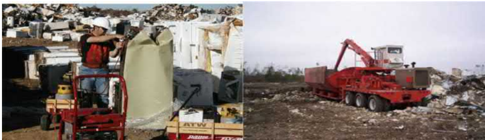
FIG. 29.3 Removal of refrigerant from refrigerators and crushing to reduce volume.
