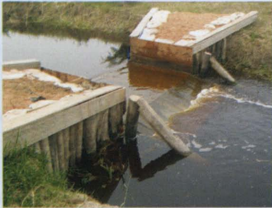
Introduction of the concept of canal blocking in Desa Bantayan, Rokan Hilir Regency
