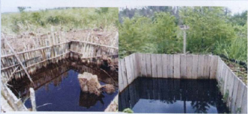
Water storage well constructed by the local communities in Desa Mumugo, Rokan Hilir Regency
