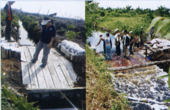
Canal block constructed using the ' spillway ' design
