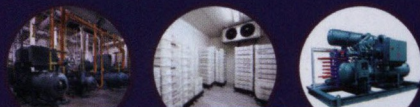
Large Pumped System Small / Medium DX Chiller + Secondary Fluid 50 to 5000 kg 10 to 100 kg 100 to 2000 kg
