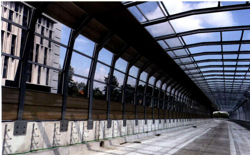
Figure E-19: Semi and partial enclosure for highway and railway noise mitigation.
