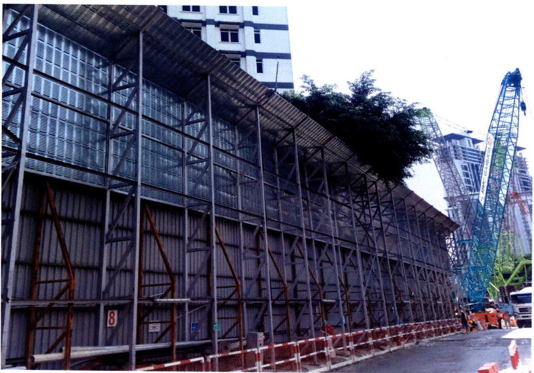
Figure E-10: Temporary noise barriers used in MRT construction noise mitigation
