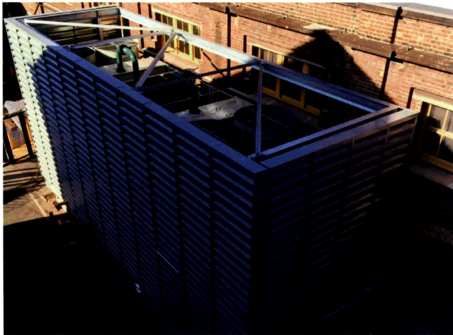
Figure E-22: Acoustic louvers used for natural ventilation opening in power station turbine hall
