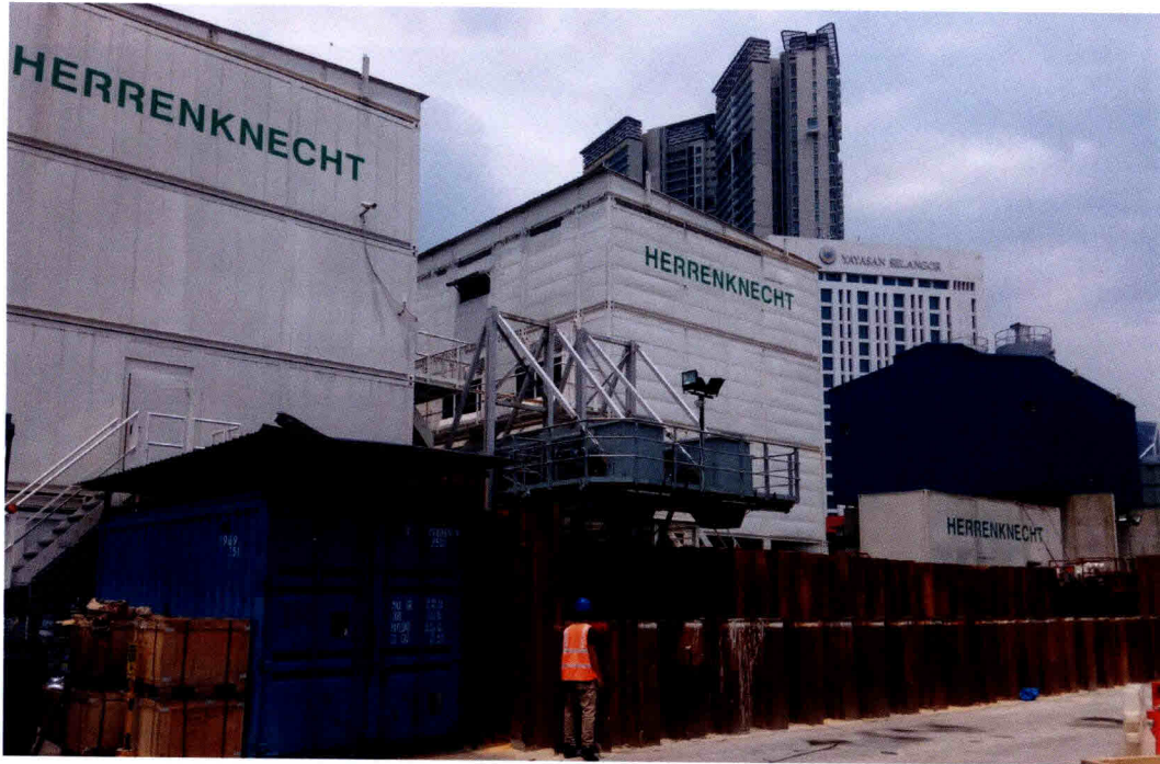
Figure E-15: Full enclosure for slurry treatment plant in Klang Valley MRT construction work site adjacent sensitive receptors
