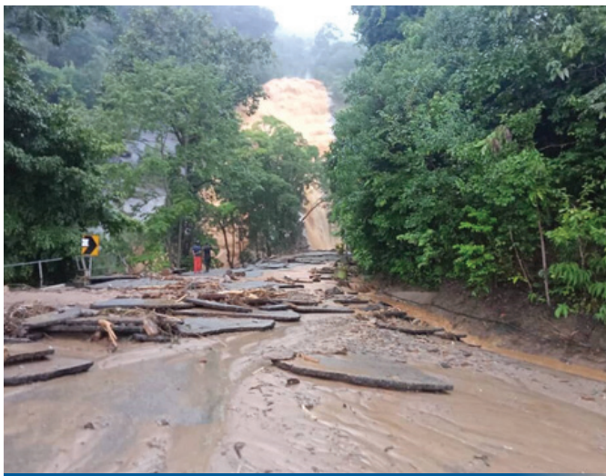
Figure 3: The Debris Flow Situation at the Disaster Location (Source: DID, 2021)
