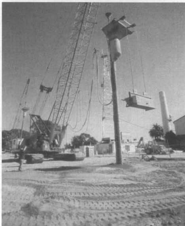
Fig. 5. Dry bottom-feed vibrocompaction using stone backfill
