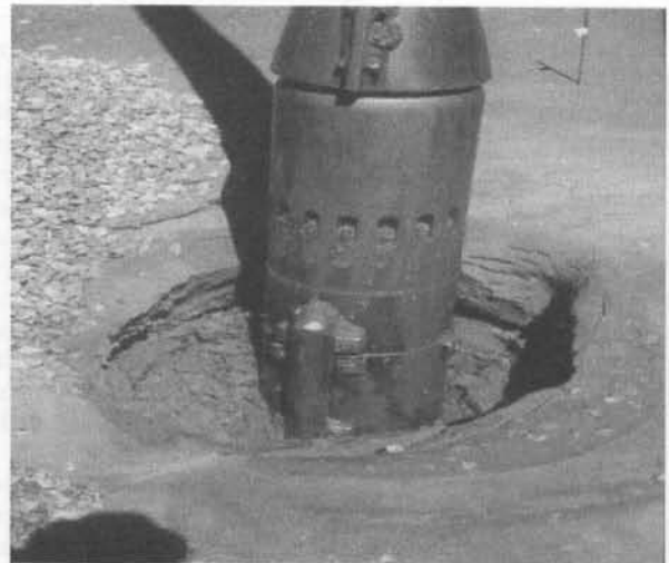
Fig. 4. Wet vibrocompaction during the compaction phase
