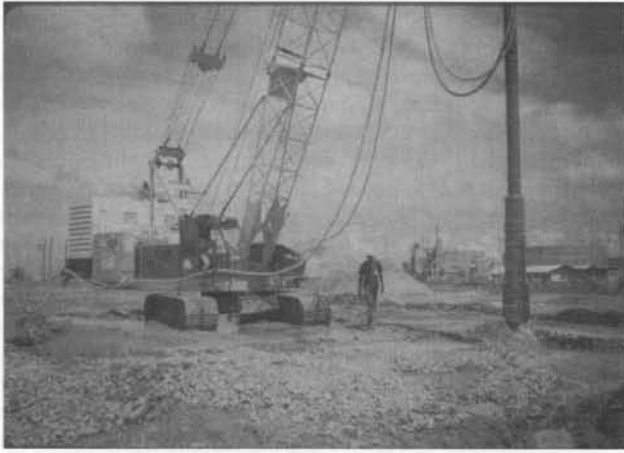
Fig. 2. Wet vibrocompaction plant ready to commence
