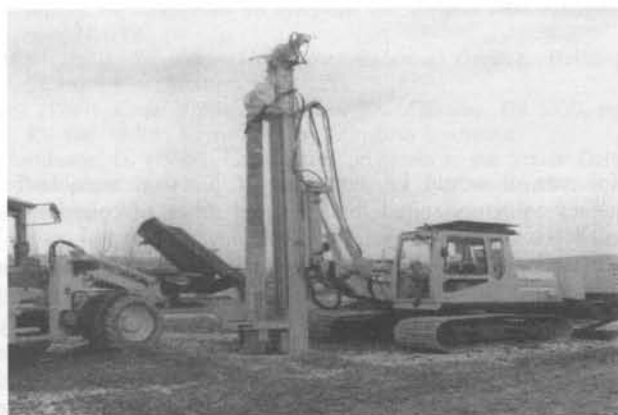
Fig. 10. Purpose-designed small-scale plant for vibrated stone column construction
